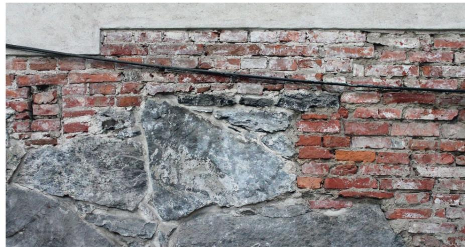
Image 9. Artilleristallarna today. Tactile materials where the wall meets the stone masonry foundation.
