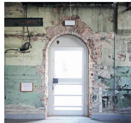
Image 27. A former window, converted to a door in the former northern stable. (Wallenstam, 2018) Adapted with permission.
