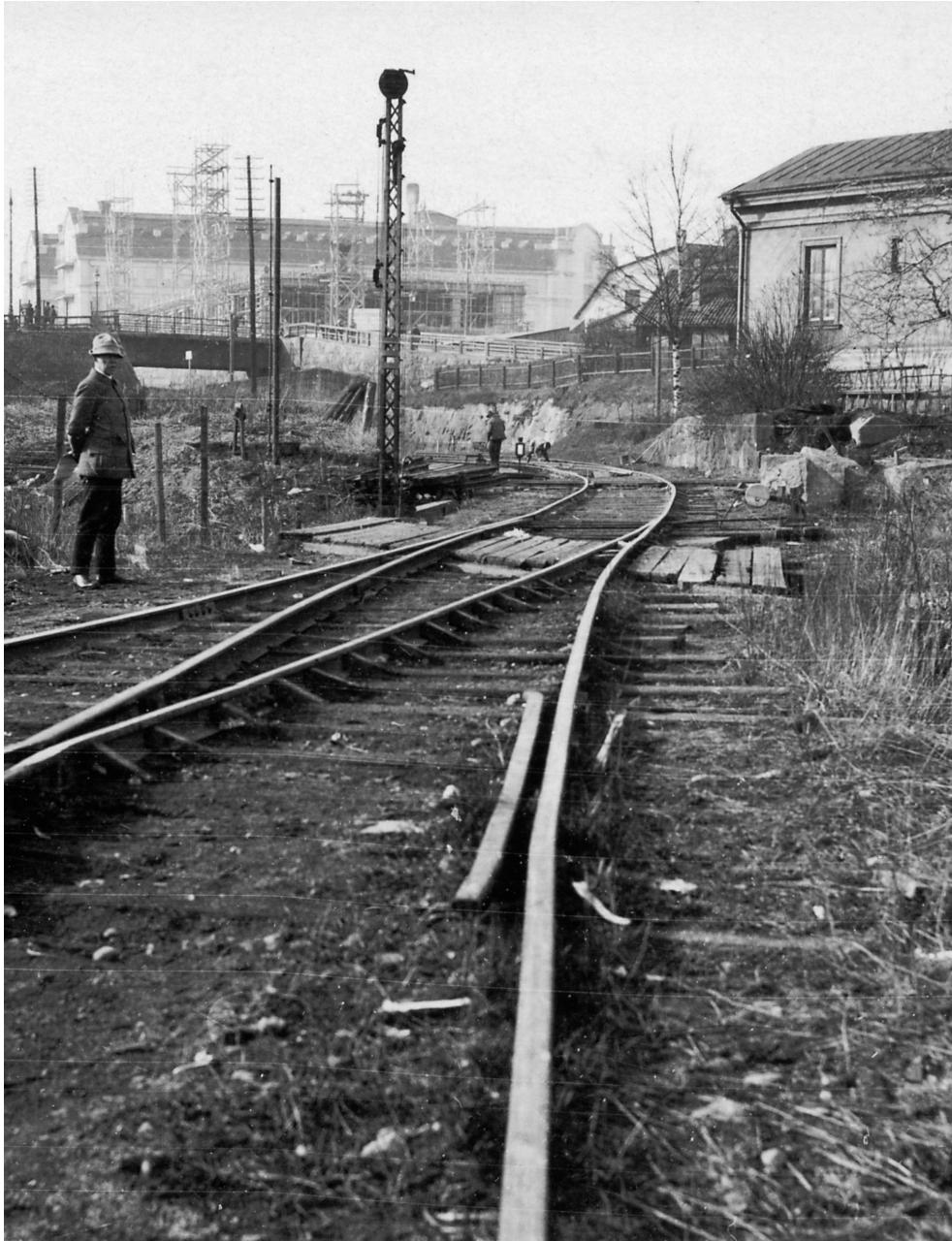
Figure 7. In process of building the warehouse (Järnvägmuseet, 2019).
