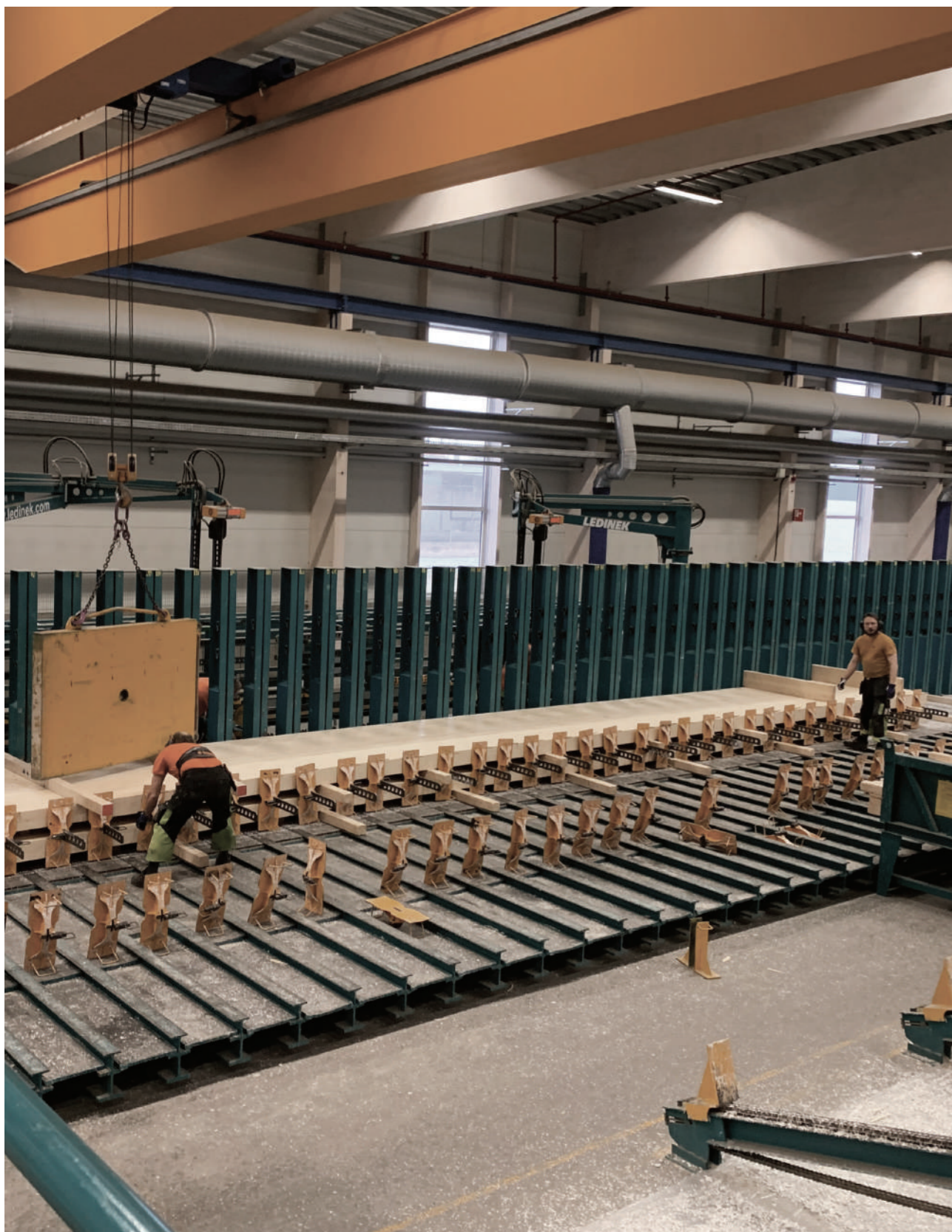
Robot controlled clamp that can interlink lamellas into complex shaped glulams.
