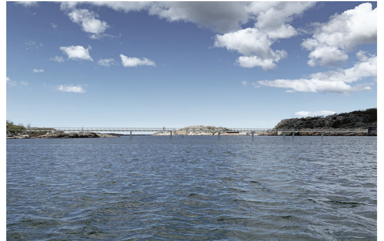
Entire bridge seen from east.
