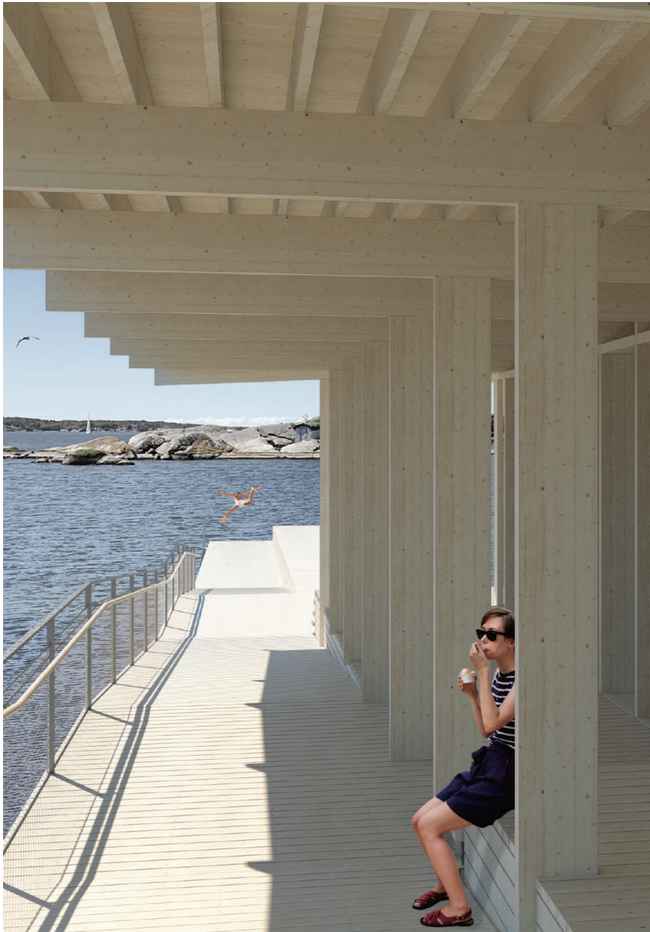
East arcade with pier ahead.
