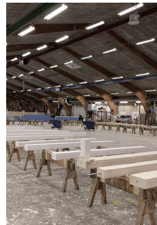
Manual working station for project specific glulams (coffee break at the time).
