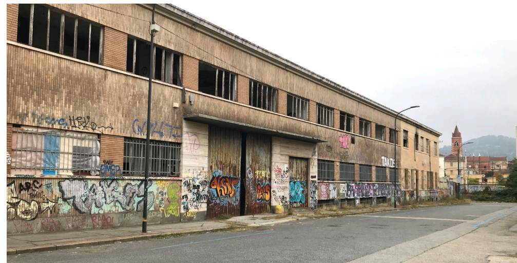
Figure 10. Current situation of Flli Miroglio building
