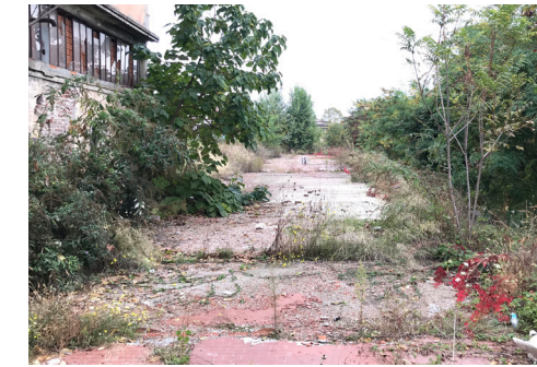
Figure 15. Foundation floor leftover
