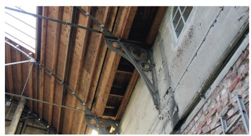
Image 8. Another characteristic feature are the slender cast iron roof trusses.
