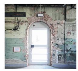
Image 27. A former window, converted to a door in the former northern stable. (Wallenstam, 2018)
