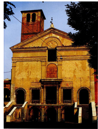
Fig37:San Sebastiano (Mantua), West Facade
