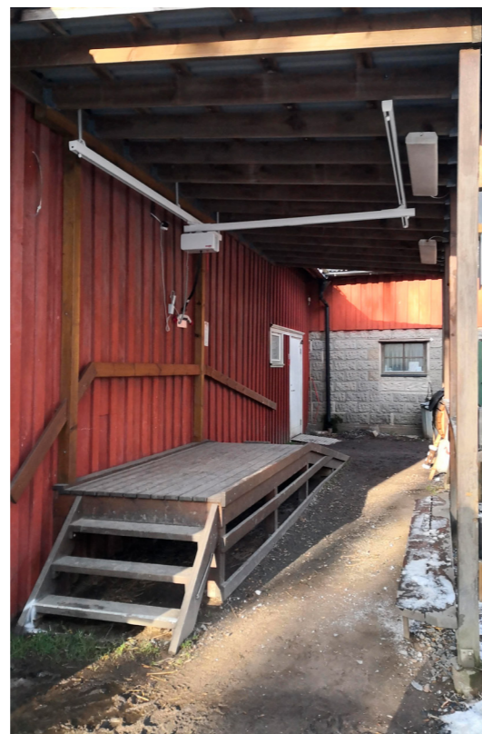
weather protected ramp with suspension system
