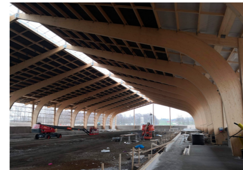
100 meters long arena with curved beams
