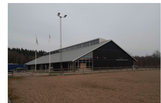
walls made of slidable elements which can be opened during the summer
