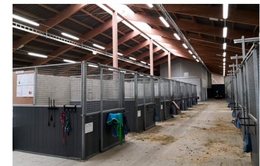
Flexible box walls which can be removed and cleaned out with a machine
