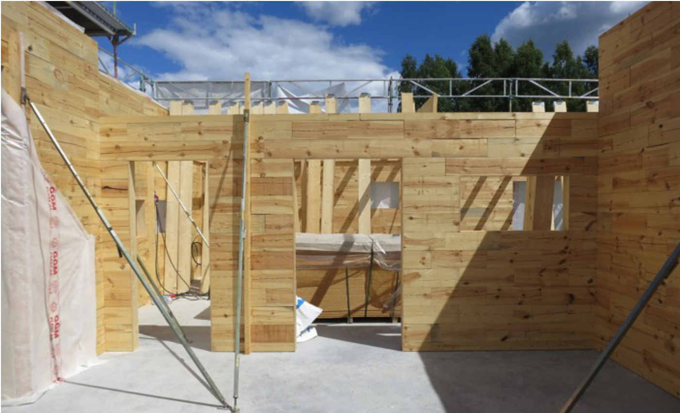
Picture 12. Bosum building system, assembling at building site, source: Bosum AB
