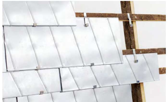
Fig. 4.26 – Facade detail - Vandkunsten , Retrieved from: vandkunsten.com/en/projects/component-reuse
