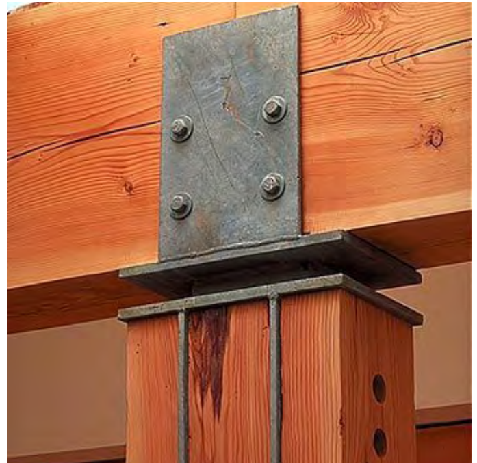
Fig. 4.11 – Heavy timber joint - Acton Ostry Architects Retrieved from: https://www.actonostry.ca/project/mount-currie-health-care-day-care/
