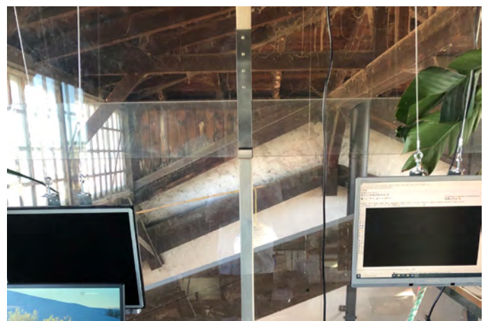
Fig. 4.43 – Upcycled security glass , Photo: Walter Unterrainer
