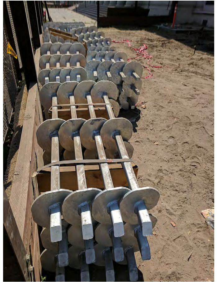
Fig. 4.05 – Helical anchors - Photo by: Argyriou, Retrieved from: https://en.wikipedia.org/wiki/Screw_piles
