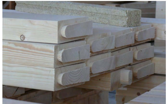
Fig. 4.16 – Geometric connection – Swallow tail - Walter Unterrainer
