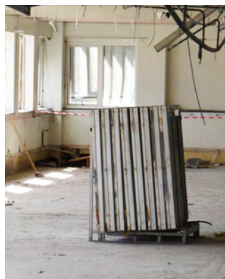
Fig. 4.33 – Demounted windows from a demolition , Own photo
