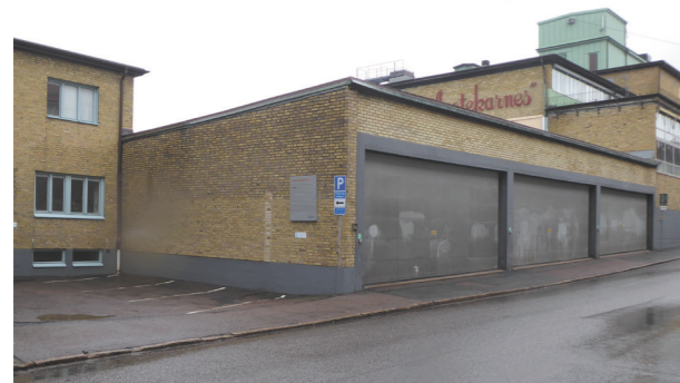
The site of the parking space and garage in its current condition.
