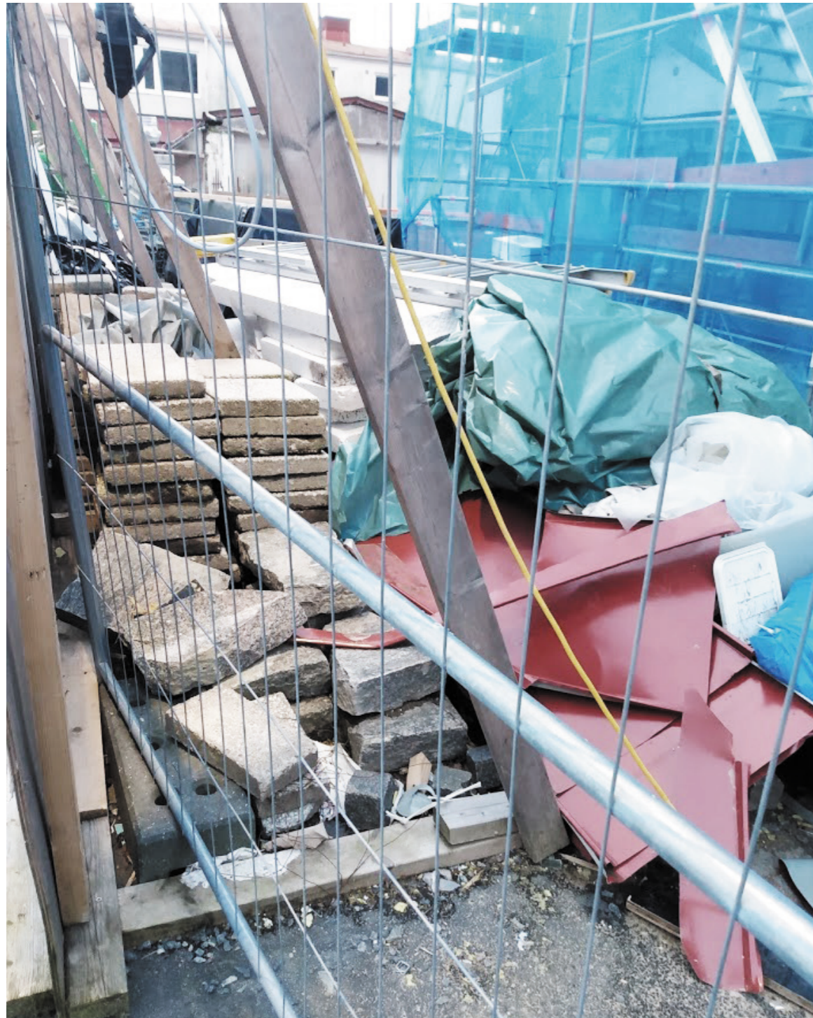
Image showing a contemporary Swedish building site.
