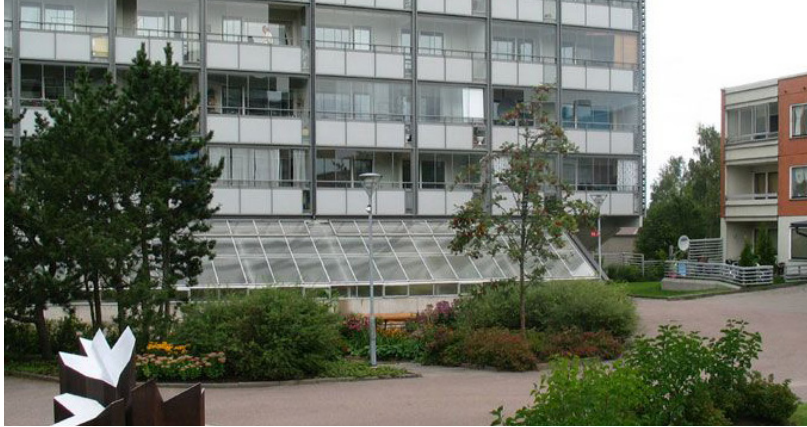
Figure 14. Solhusen in Gårdsten have combined laundry rooms and greenhouses (Nordström Kelly Arkitekter 2000).
