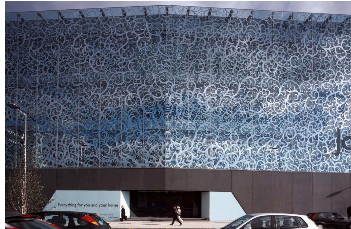
Figure 9. Facade of John Lewis Department Store and Cineplex in Leicester by FOA, (ASVL3, 2008). CC BY 3.0
