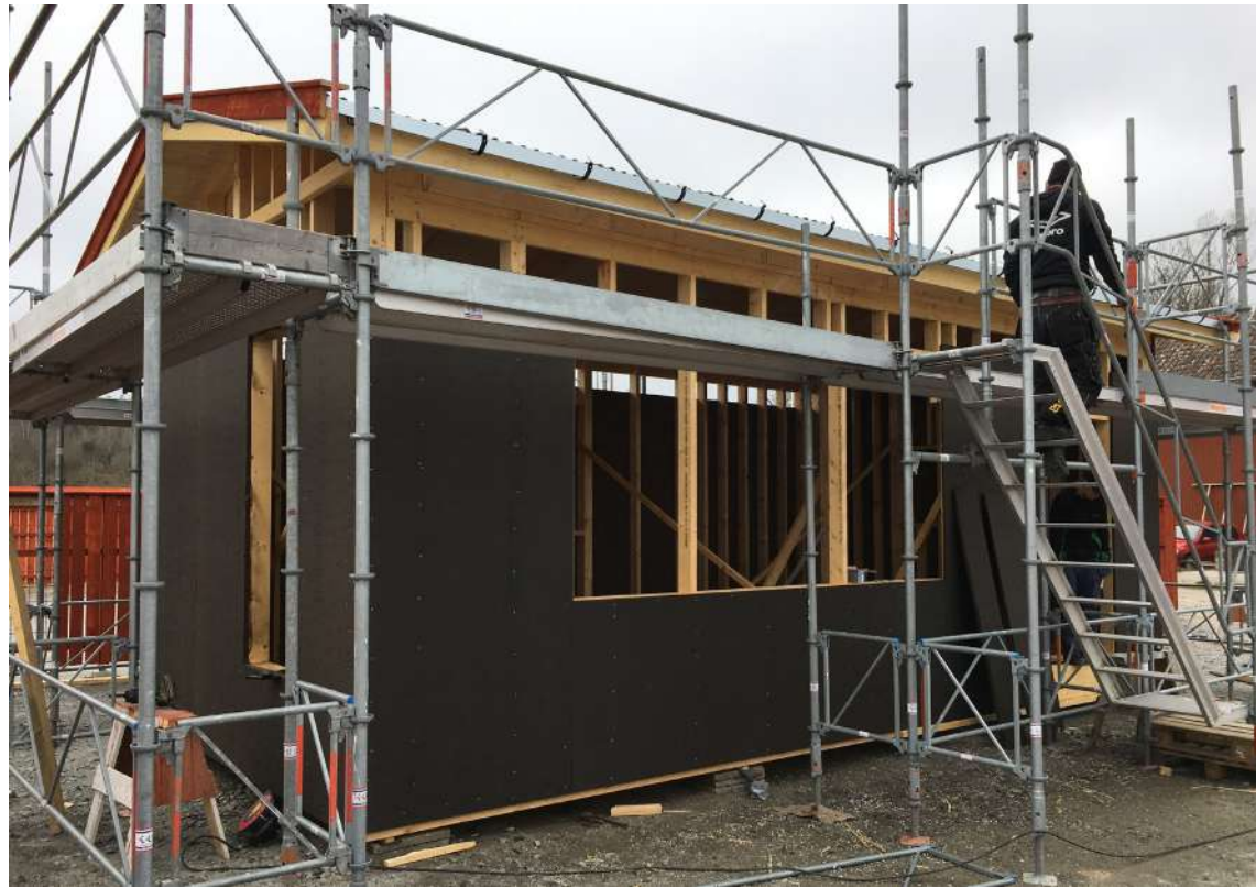
Image 71. Mounting of Asfaboard. April 15
