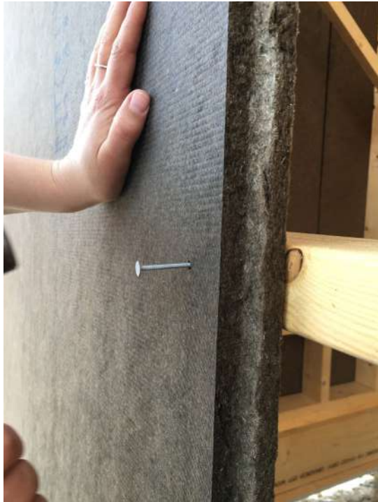
Image 70. Mounting of Asfaboard. April 15
