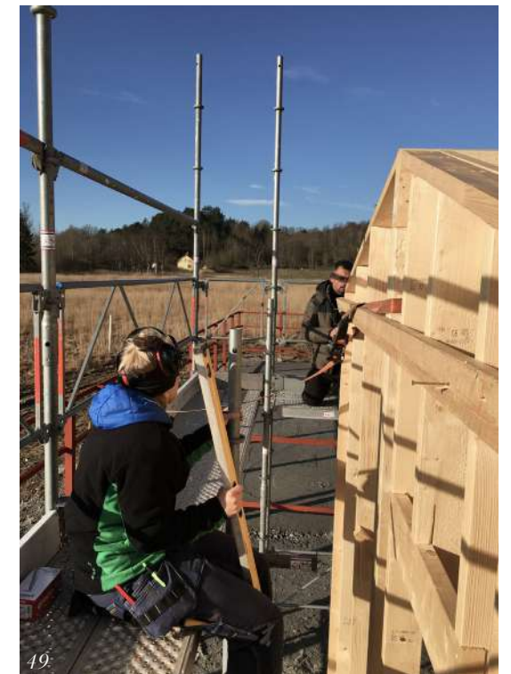
Image 48-49. The gables were straightened up with the help of one of the carpenters and because the walls were screwed together, this could be done fairly quickly. As soon as the errors were corrected, the rafters had to be remounted. April 1
