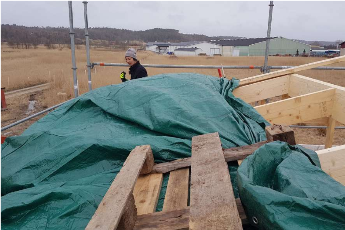
Image 53. The tongue and groove is very sensitive to wetness. A storm warning had been announced and it took 1.5 hours to secure a tarpaulin. April 1
