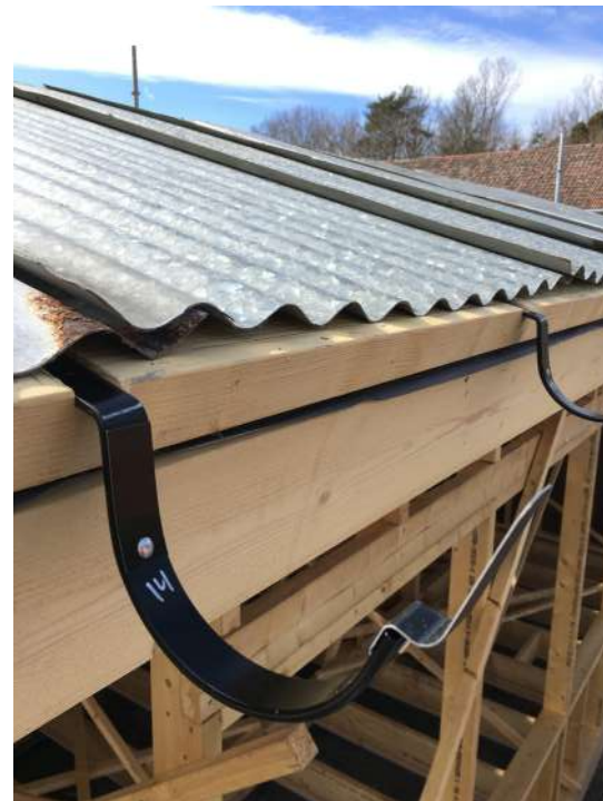
Image 64. Mounting of new gutter brackets. April 14
