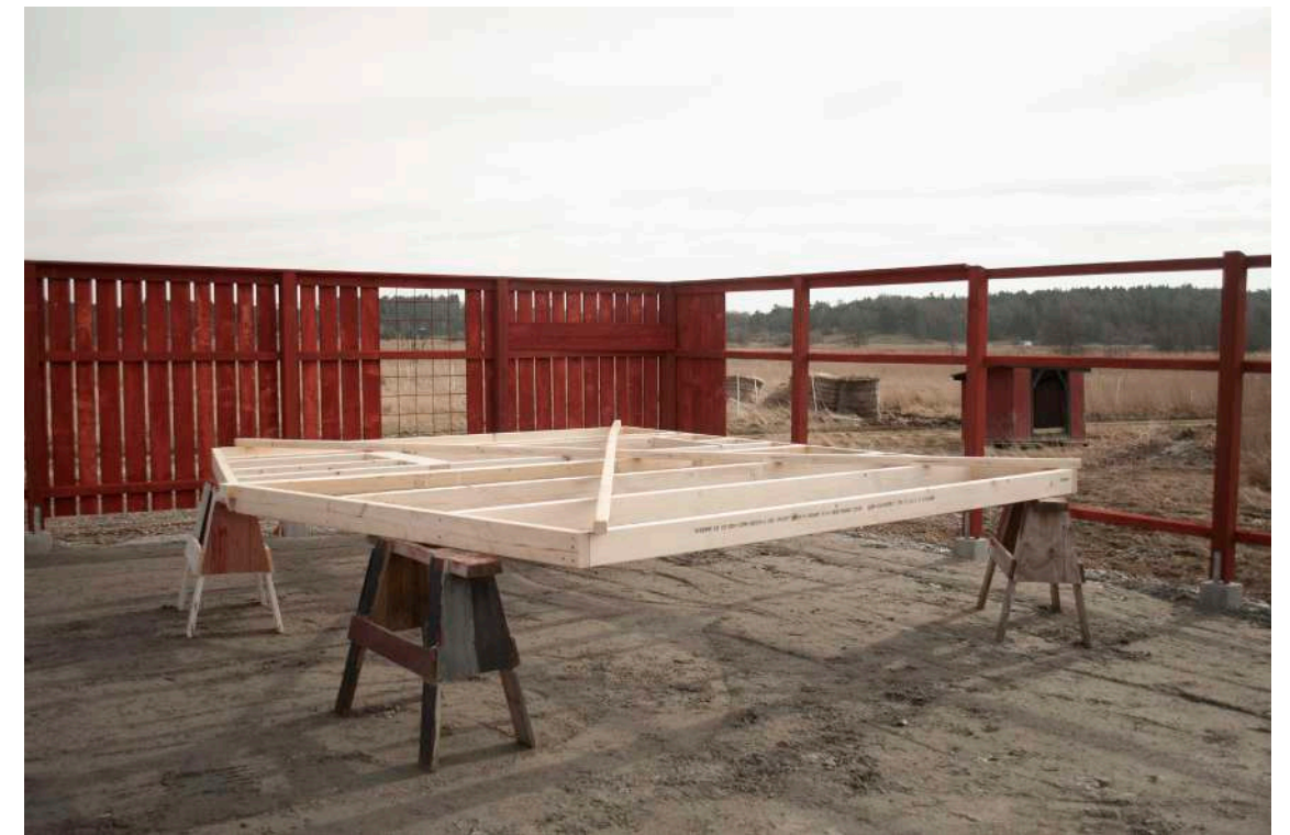
Image 35. Temporary placement of the gables. March 24
