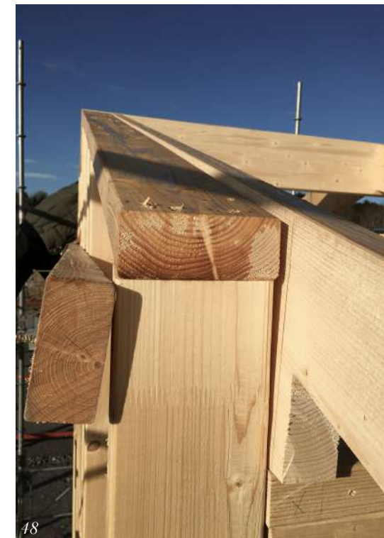
Image 48-49. The gables were straightened up with the help of one of the carpenters and because the walls were screwed together, this could be done fairly quickly. As soon as the errors were corrected, the rafters had to be remounted. April 1
