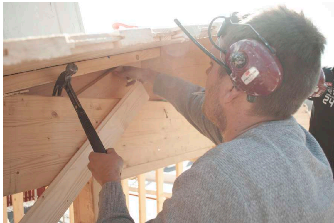
Image 55. Carpenter fixing the flying ridge beam. April 6
