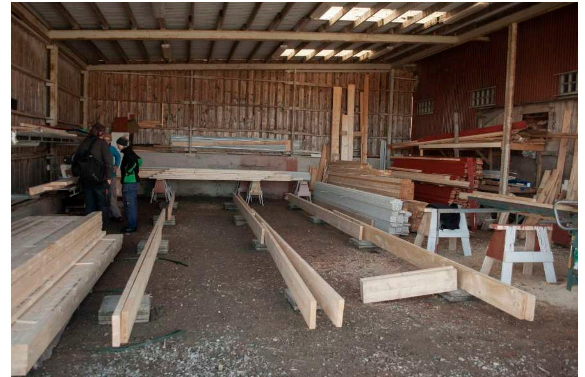
Image 23. Start of the floor structure. March 11
