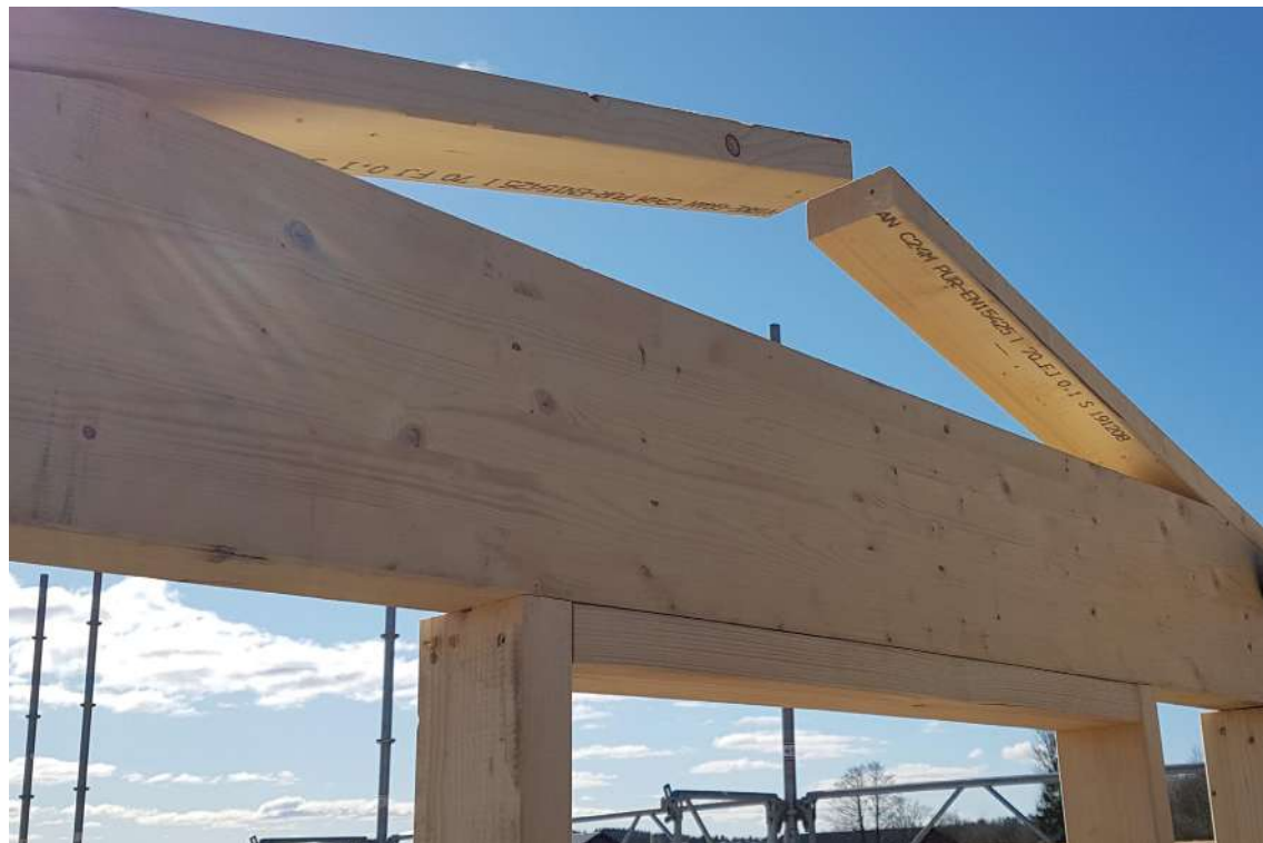
Image 45. Mounting of the unloading beam which was sawn from the ridge beam. March 30
