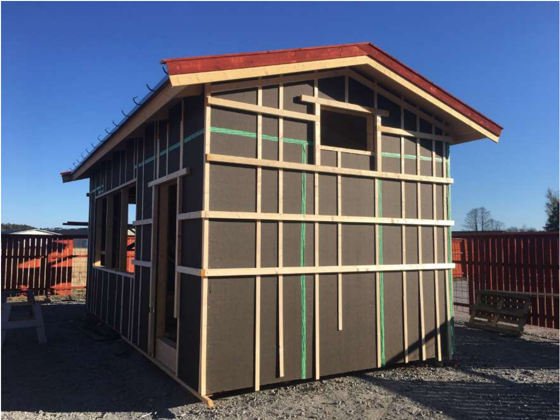
Image 74. Wooden battens mounted on the asfboard. April 22
