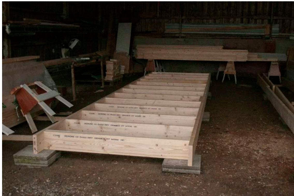
Image 24. First half of the floor structure. March 11
