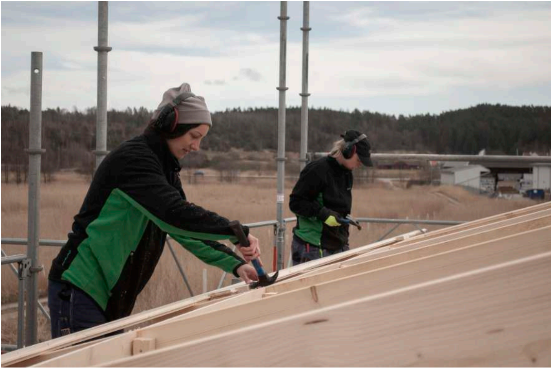
Image 52. Mounting of tongue and groove. April 1
