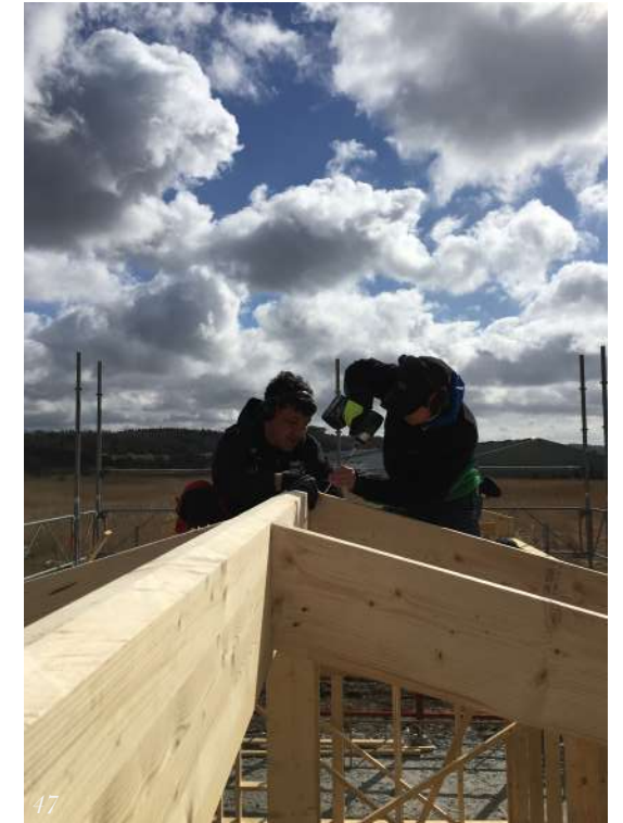
Image 46-47. When the ridge beam was mounted on the two gable walls and the rafters were mounted on the beam, an error was discovered. The two gables were askew, making the rafters too long for the house causing them to fly in the air. March 30
