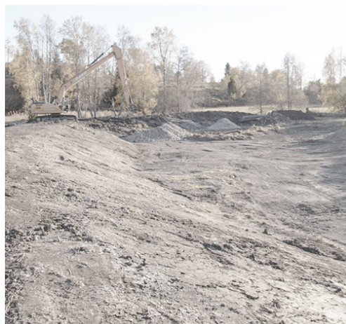
Newly constructed soil Embankment (Söderman, 2018)
