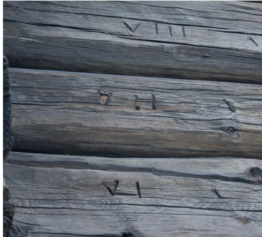
"skvaltkvarnen" at Gammelgården shows markings to keep track of the pieces when the building is disassembled and put together again
