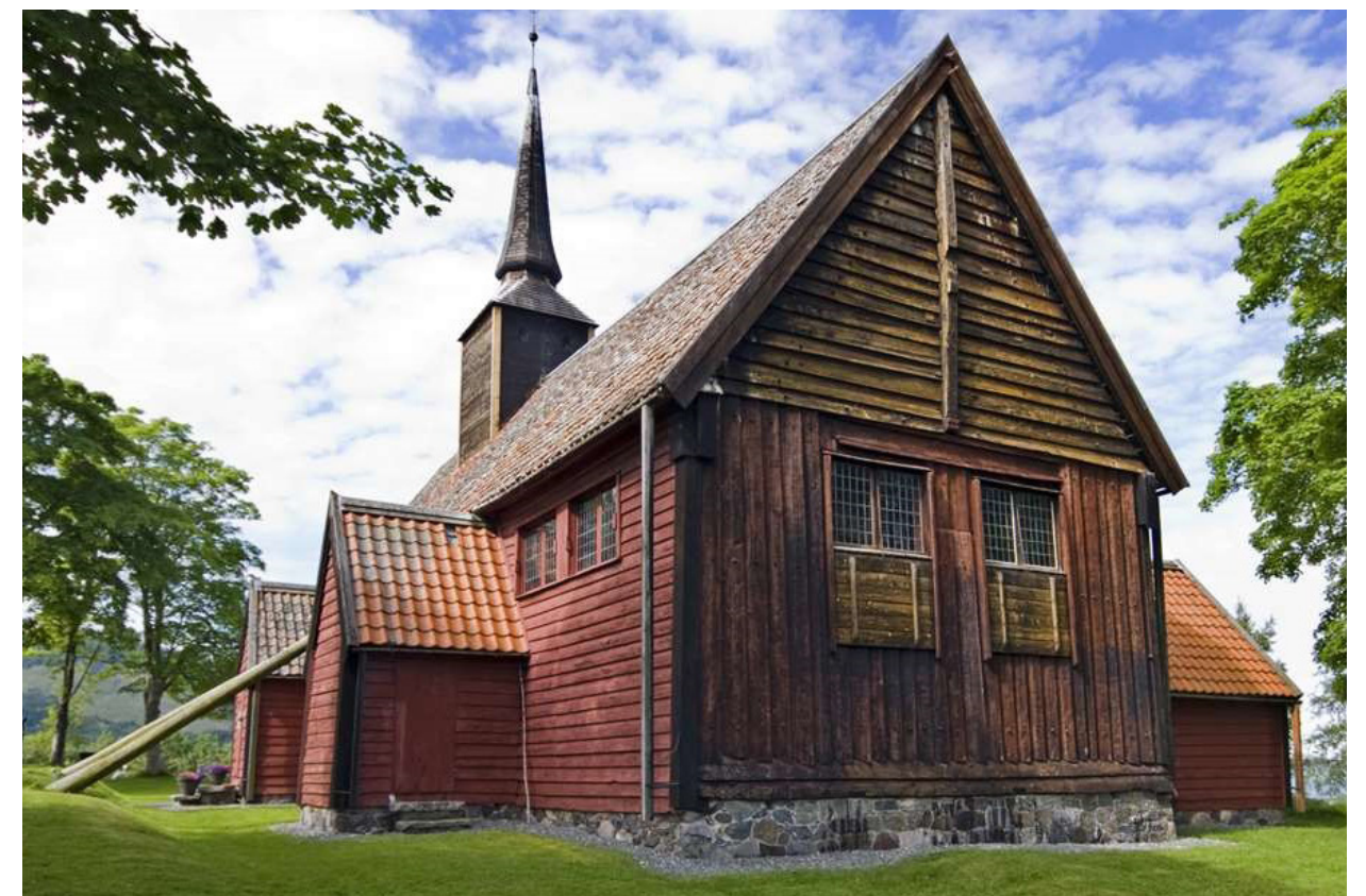
Fig.6 Wooden cladding of Kvernes stave church built in the 17 th. century in Kvernes, Norway. It is one of the oldest claddings in the Norway. (Godal, 2012)
