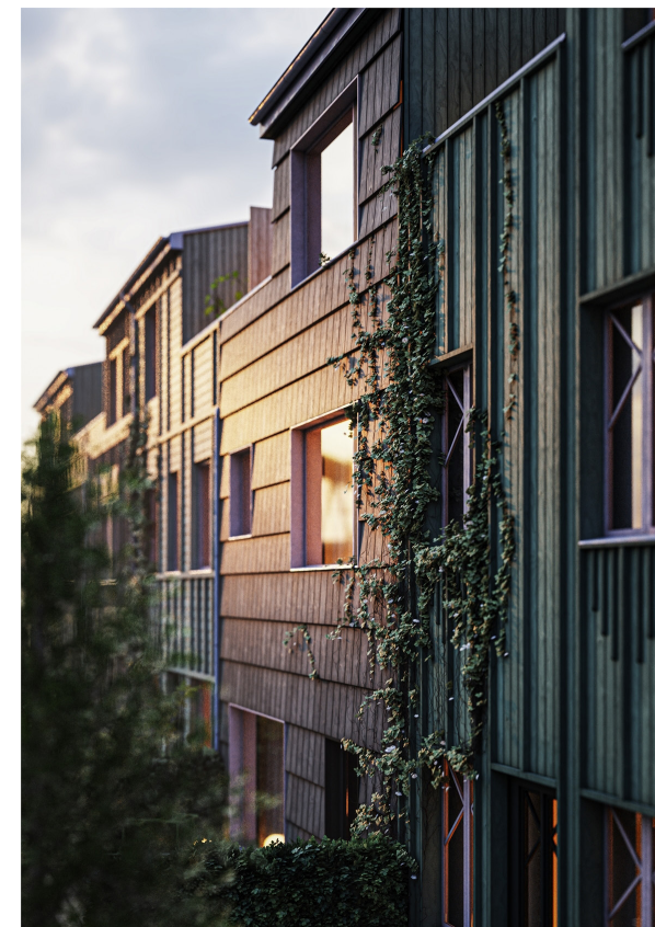
Fig.40 The images above show the different cladding solutions in the south facade,
