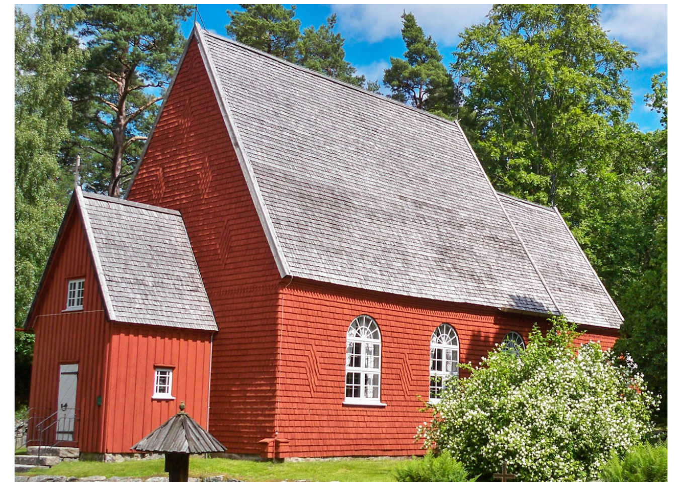
Fig.38 Southwest view of the of Ramna church. The walls are covered with church shingles that are treated with red slamfärg.
