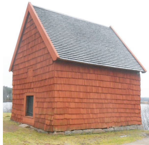
Fig.11 Ingatorp tithe barn in Sweden, its shingle cladding is a protective layer that shelters the log walls (Melin, 2019). More information is shown in the case study section.
