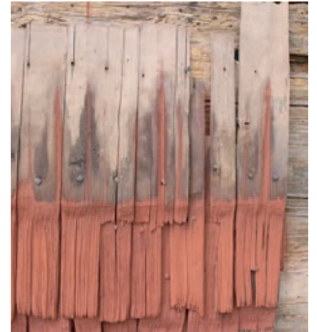
Fig.33 Restoration works of the cladding. The shingles are nailed directly to the log walls.
