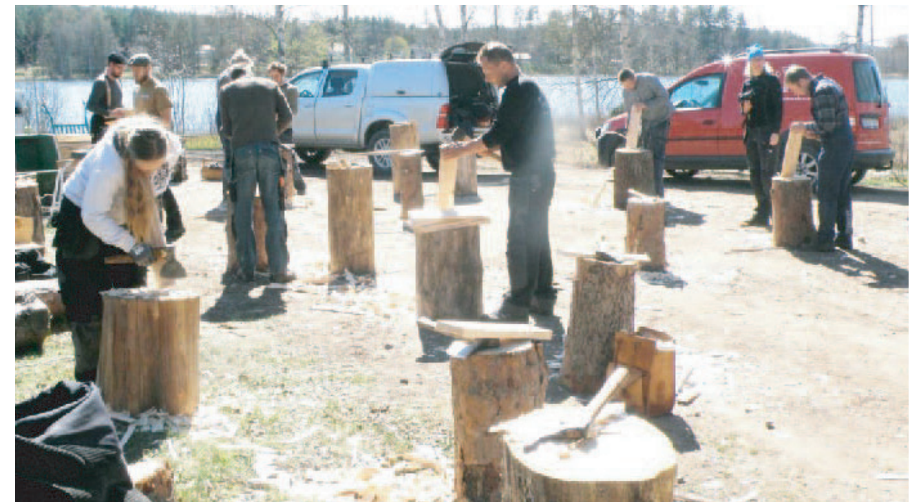
Fig.34 Ingatorp thite barn restoration project, the image shows the making of new chopped shingles. 400 new shingles were crafted in a shingle seminar in 2014.
