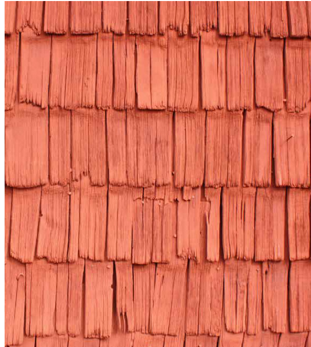
Fig.31 Ingatorp thite barn shingle wall. The shingles are placed edge to edge horizontally and they are overlapped vertically.
