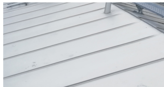
Roof tin sheets on the existing roof.
