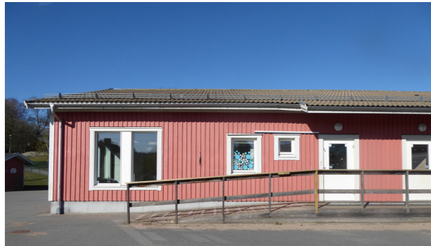
Facade of Biskopsgatan 8.
