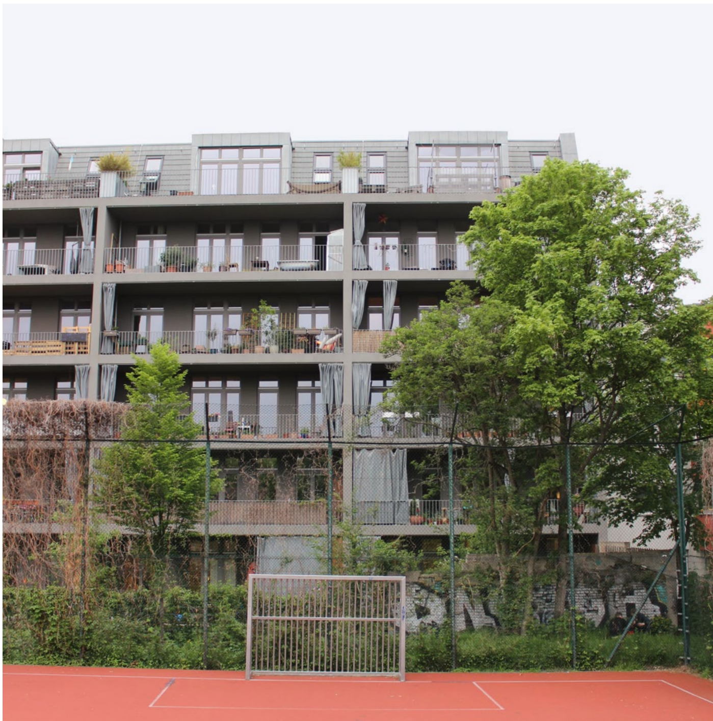
Figure 11: Ausbauhaus Neukölln, a contemporary example of a joint building venture in Berlin.
