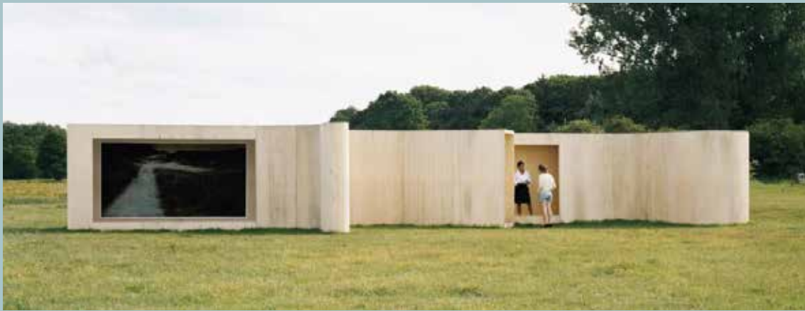
Fig. 4 Temporary Museum by Anne Holtrop
