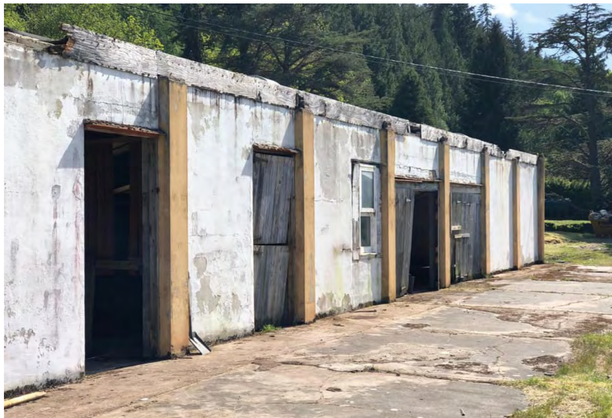
Fig. 4 Front view of the Piggery. Reprinted with permission.
