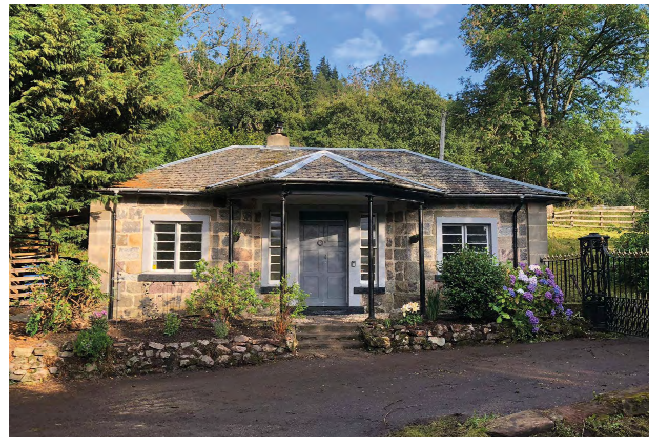
Fig. 5 Front view of the Gate Lodge, with iron gates on the right side. Reprinted with permission.
