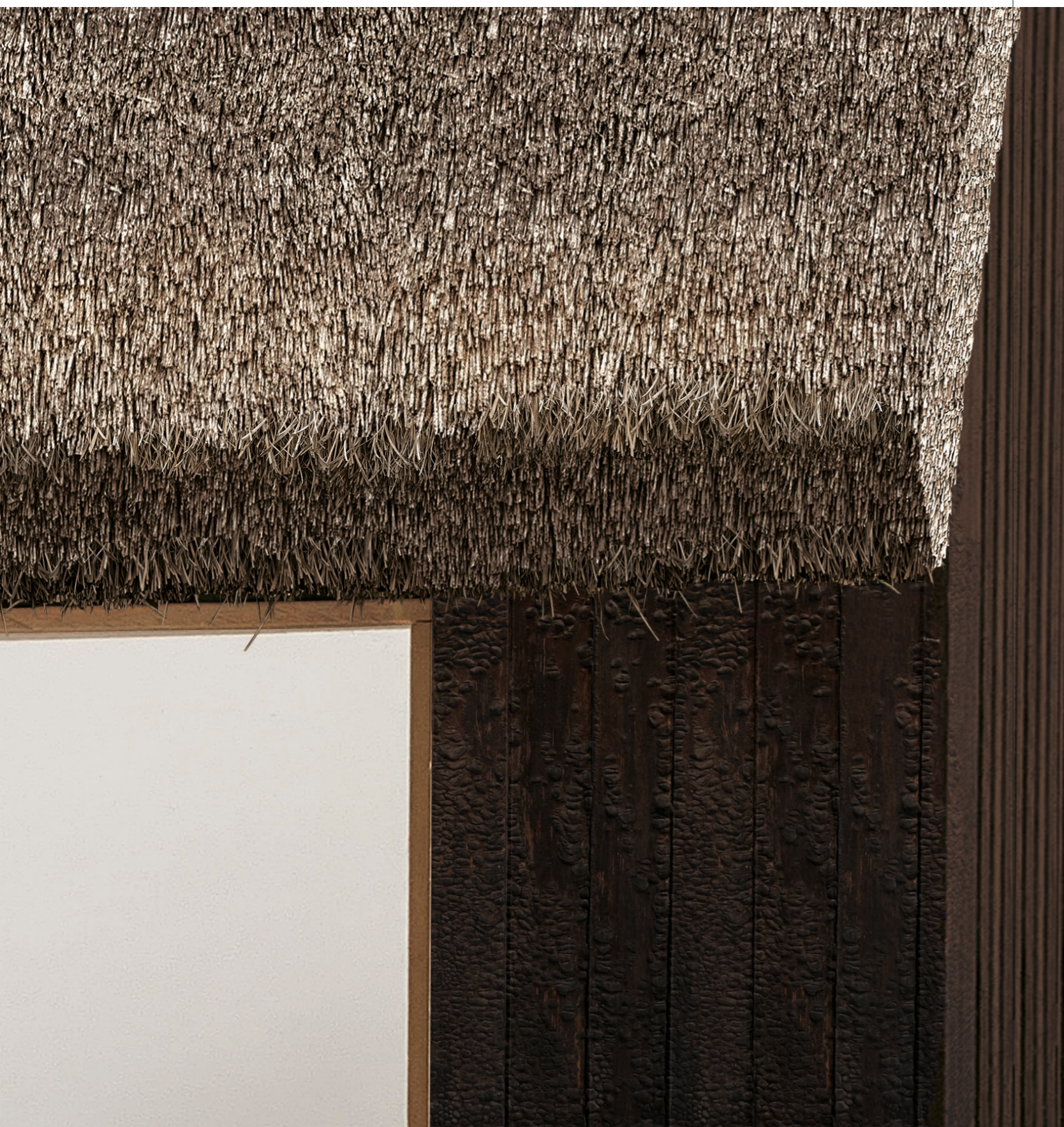
Old tar will get wrinkled drop-formations after generations of tar layers. This can be scraped off or kept as a sign of age.
