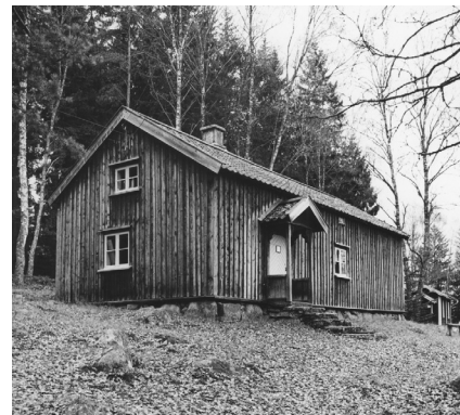
Figure 10. Wooden cladding to protect the timber structure (Björnånger, 2015). CC BY-SA
