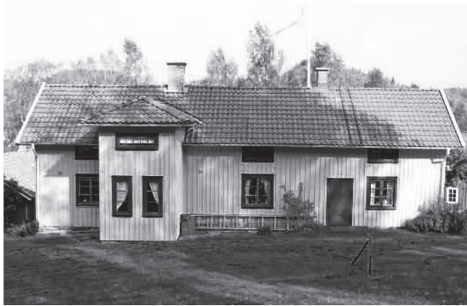
Figure 15. Unheated extension concept of a vernacular Framkammarstuga. The entrance to the heated part of the house works as a buffer zone (Hansen, Nordström, 2007).
