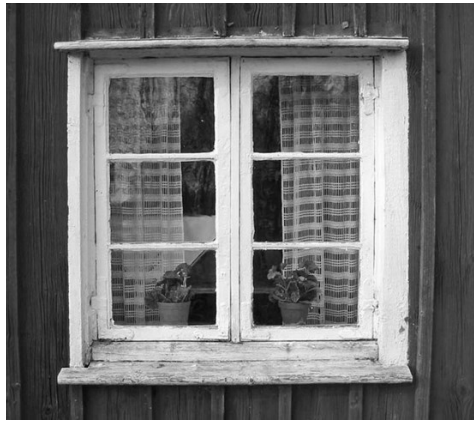
Figure 13. Single glazed window with interior winter pane. Air is warmed between the panes before it enters the dwelling (slöjd och byggnadsvård, 2021)
