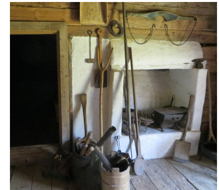
Figure 9. Horizontal timber structure with granite stove. (Franzén, 2018).
