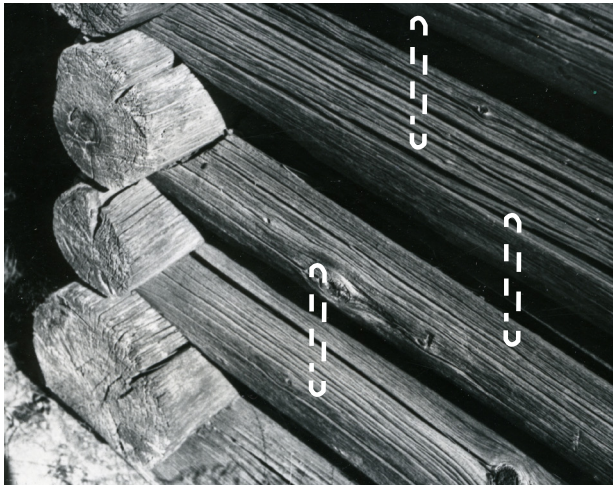
Figure 16. Traditional timber wall with internal wooden dowels (Västmanlands museum, 2018).
