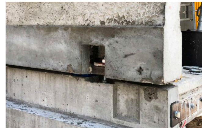
Fig 10. Picture, Circle house concrete detail. © GXN.
