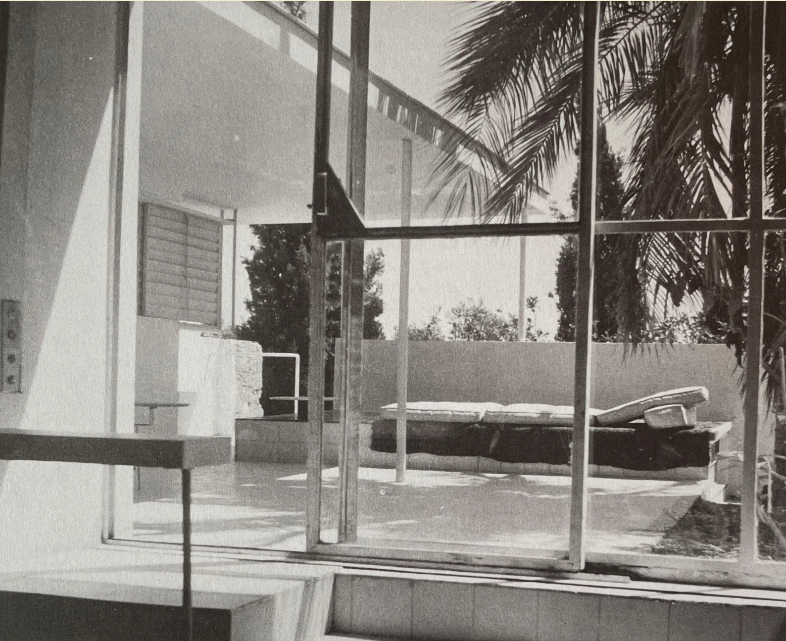
FIG. 15 / TEMPE A PAILLA, CASTELLAR / TERRACE VIEWED FROM THE LIVING ROOM/STUDIO
