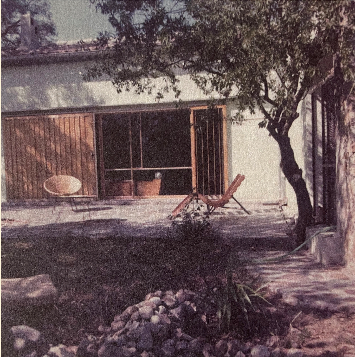
FIG. 17 / EILEEN GRAY / LOU PÉROU, SAINT-TROPEZ / SOTHERN FACADE VIEWED FROM GARDEN, WITH OUTDOOR FURNITURE FROM TEMPE A PAILLA
