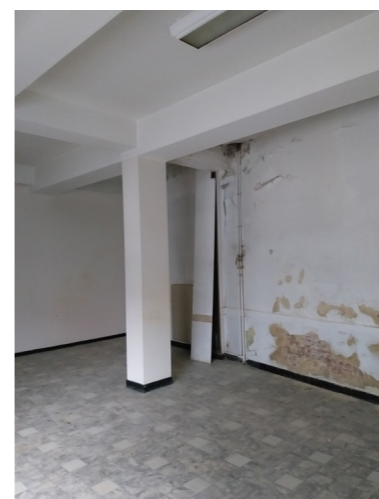
Figure 44. View from inside
