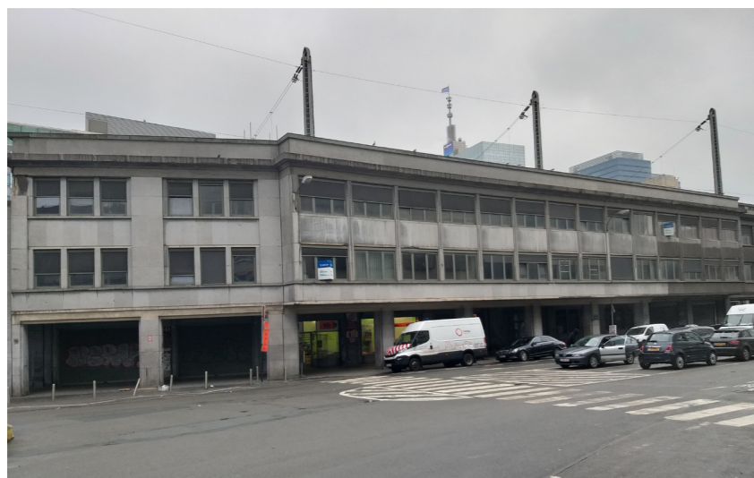
Figure 36. Building view from the South-East
