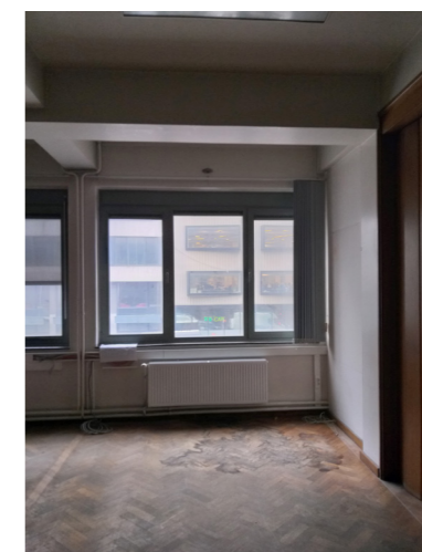
Figure 45. View from inside
