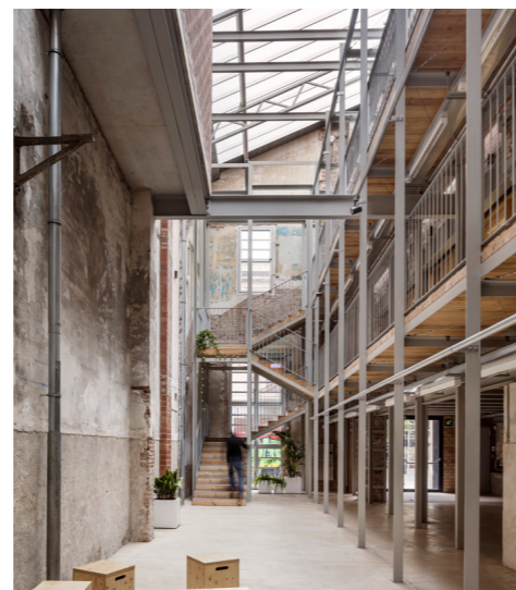
Figure 26. Civic centre view from inside (Goula A.)
