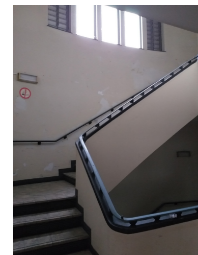
Figure 46. View from inside
