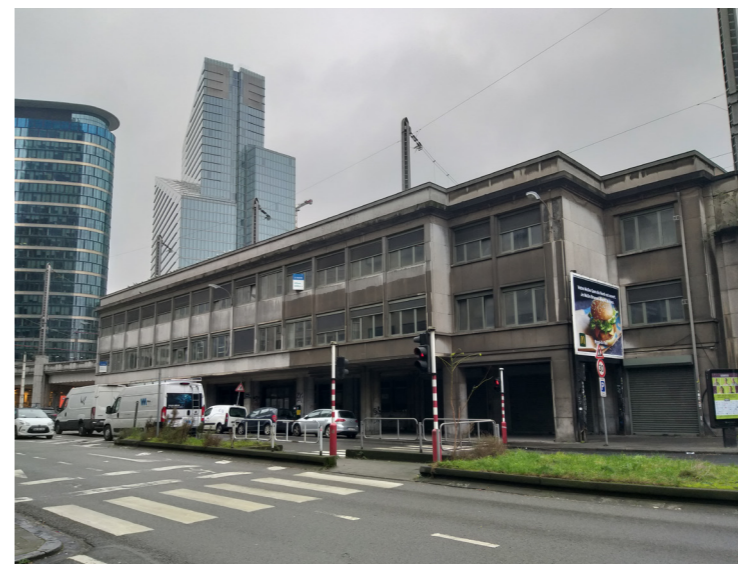
Figure 40. View from the North-East
