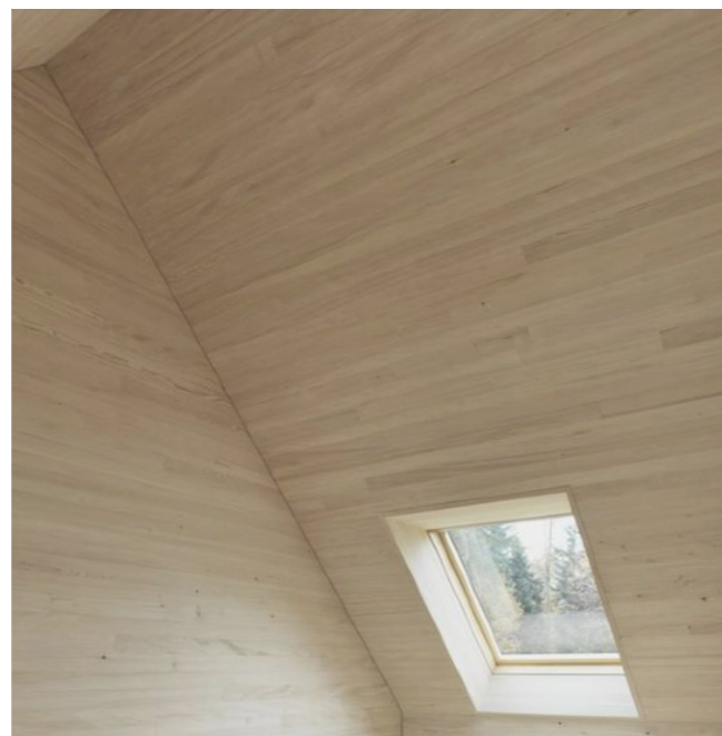
Figure 5. Airtightness makes the CLT construction perform well as a low energy and passive house (Von Radina, 2014)
