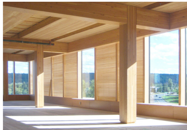
Figure 28. A way to allow exposed wood is to make posts and beams overly dimensioned and install a sprinkler system. (Archtonic, n.d.)
