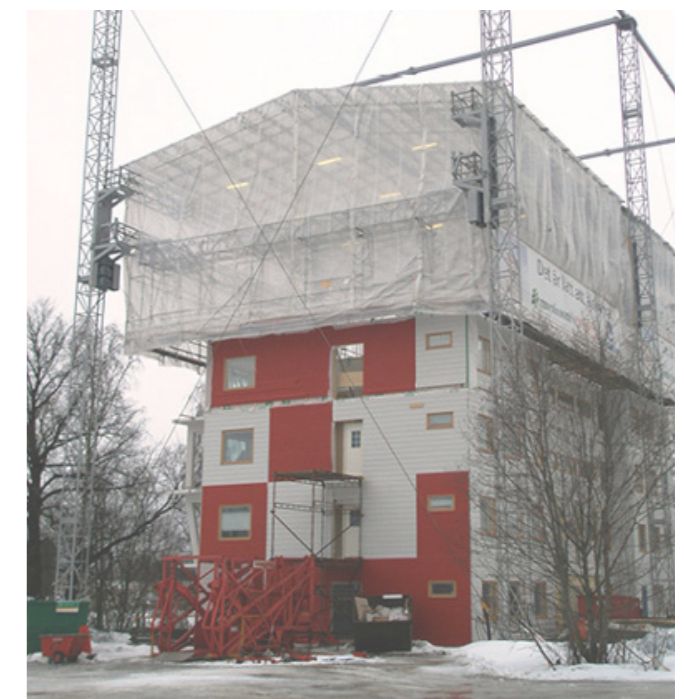
Figure 7. A weather protection on the building site can ensure a moisture free construction and give a shorter construction time. (Svenskt Trä, 2017)
