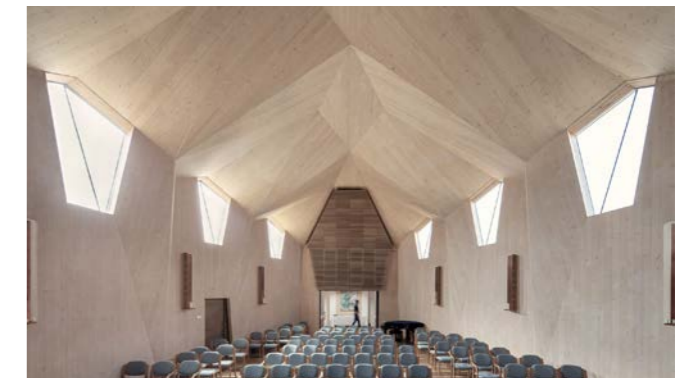
Figure 30. The chapel from Nicolas Pople Architects is a great example of how CLT-slabs can form a folded plate structure with a large span without beams or pillars. (Deezen, 2020)
