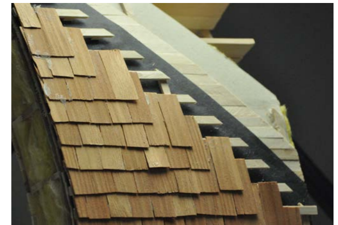
Glulam arch with shingle panel
