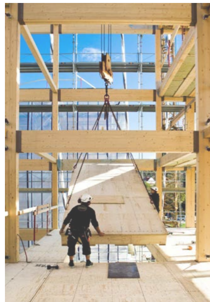
Figure 24. Post-Beam - Housing Project (Moelven, 2012)
