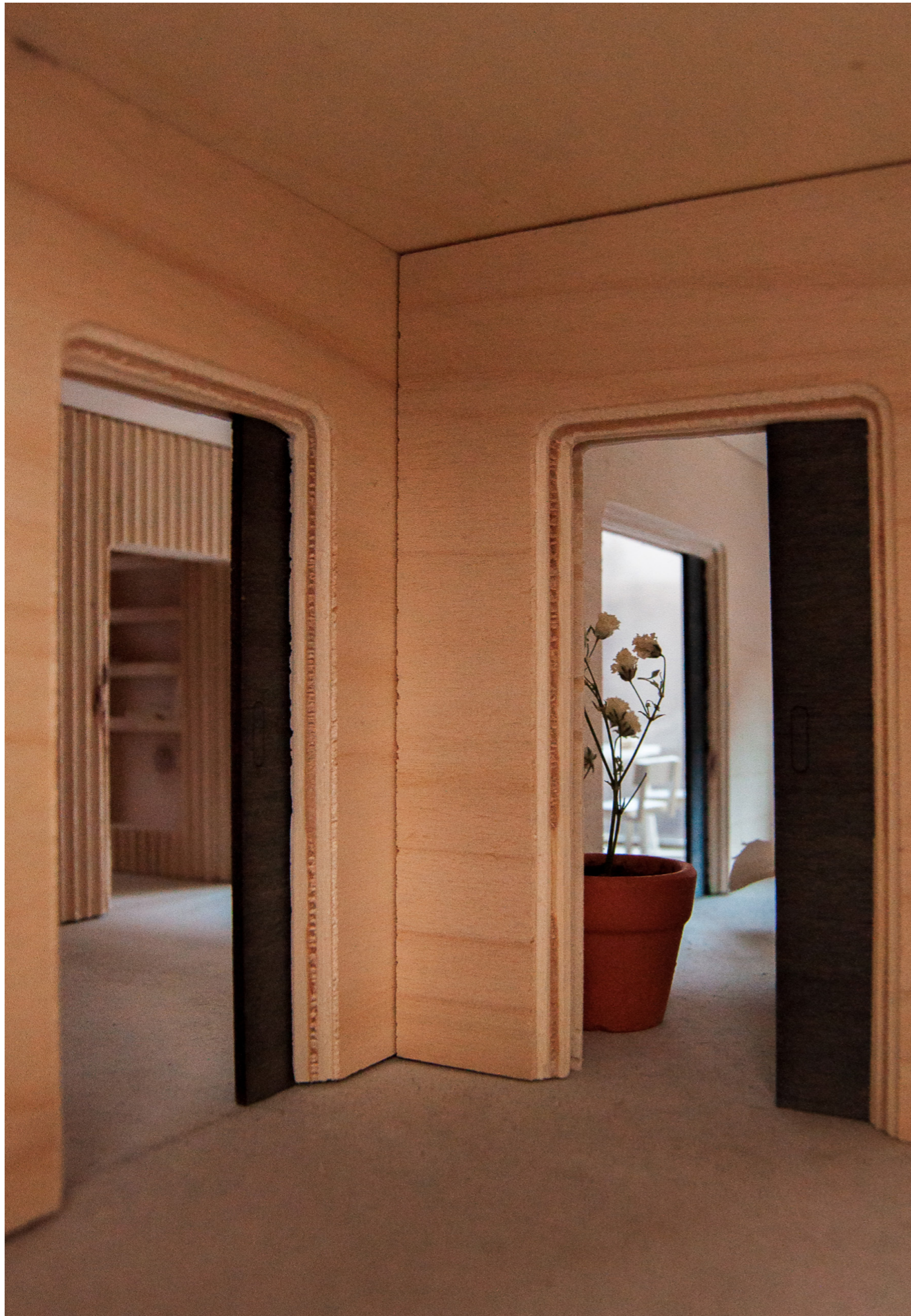
View from the hall, sliding doors are placed between the two CLT-slabs that forms the load bearing interior walls
