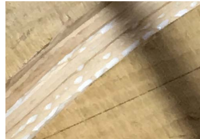
Glulam beam in form press.
