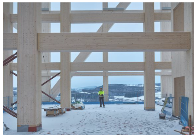
Figure 29. The structural system of Mjöstornet, the tallest wood structure in the world, is composed of glulam Posts and Beams, with lateral stability from glulam trusses (ArchDaily, 2018)
