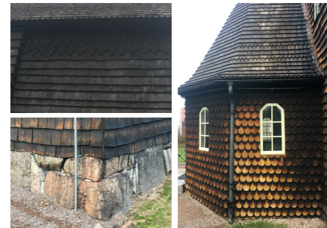
Left: Accentuated plinth and soffit. Right: Patina of facade depending on how exposed the surface is.
