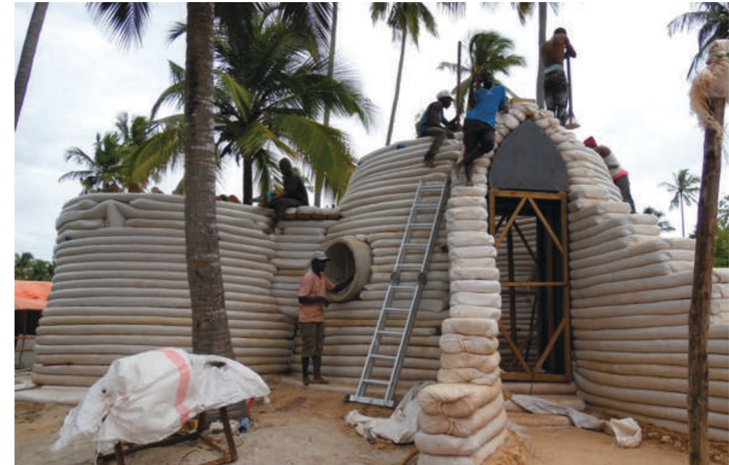
Construction of an earthbag house (Photo: California Institute of Earth Architecture, n.d.)
