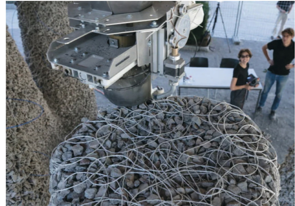
In situ robot depositing string (Photo: Christian Beutler, 2018)
