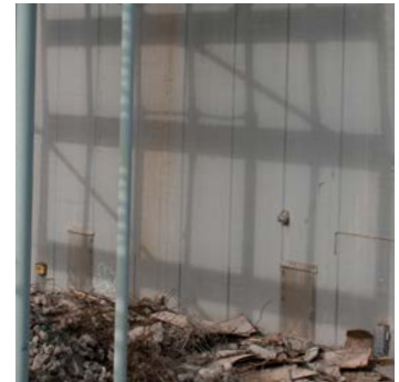
Material: Reinforced concrete and plywood Tool: Excavator and magnet Traces: Large chunks of crushed material
