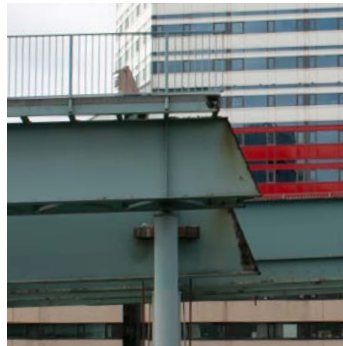
Material: Thick sheet metal Tool: Cutting tool Traces: Tilted edge with burnt gradient
