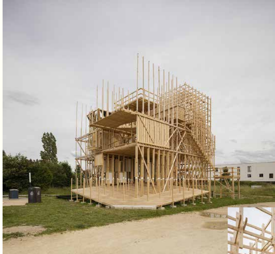
House 1 / ALICE studio architects
