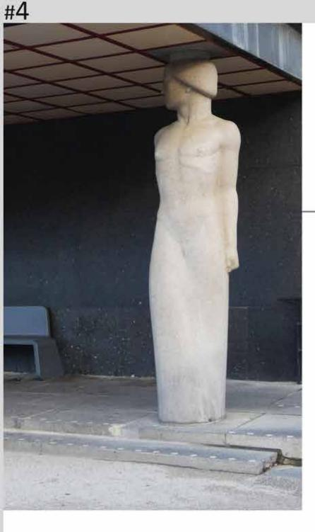
One of the unique features of Götaplatsen is the two statue/columns bearing the load of the roof covering the entrance of The City Theatre. The twist of the statue inspired a brick block to explore the curves that would be created with the possible compositions of this twist.
