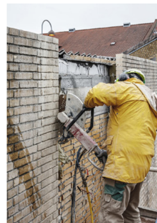
Fig. 12, Sawing out brick modules from the old Carlsberg brewery in Copenhagen
