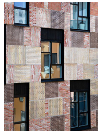
Fig. 10, The reused brickwork facade of the Resource rows
