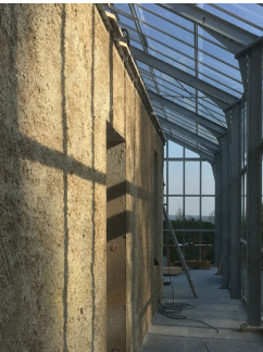
Image 28. Drying of wall
