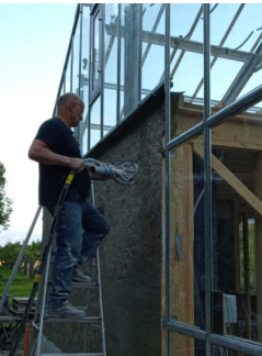
Image 27. Spraying the hempcrete
