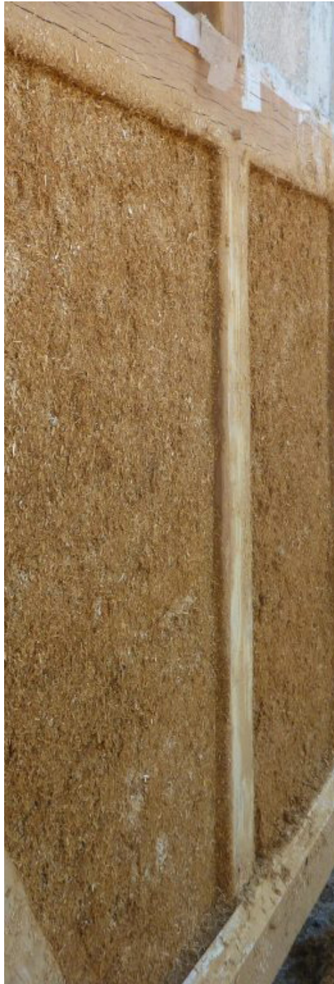
Image 48. Hemp-clay wall sprayed-applied
