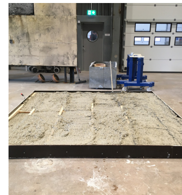
First layer of hempcrete is placed, nicely tamped and fitting around the wood.
