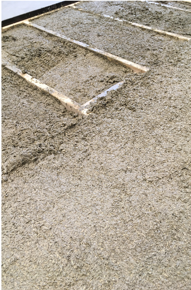
Image 1. Hempcrete in wooden formwork
