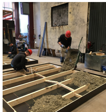
The mixture is poured in the framework.
