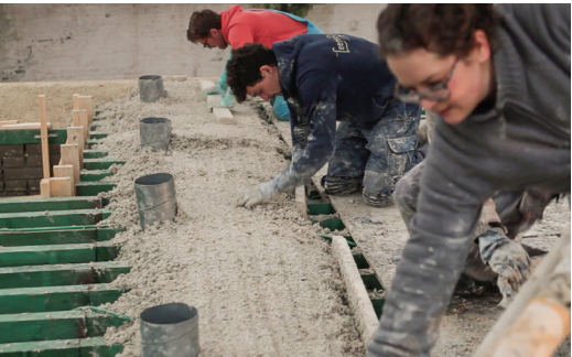
Image 31. Placing hempcrete on the roof
