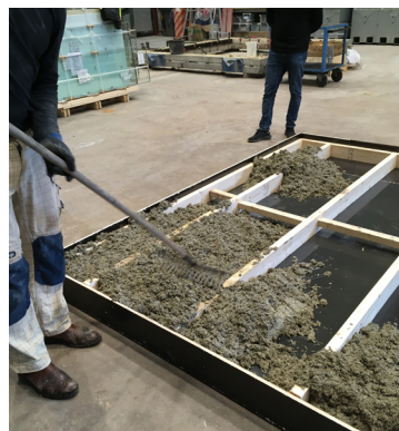
It is spread, pushing it onto the wood to remove air in every corner.
