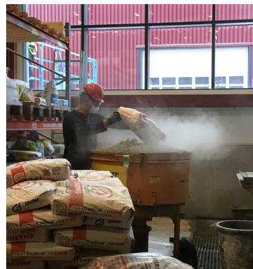
Pouring 2 bags of lime binder in the mixer (2x18kg).
