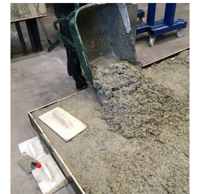
New batches of hempcrete are added to form a second layer.
