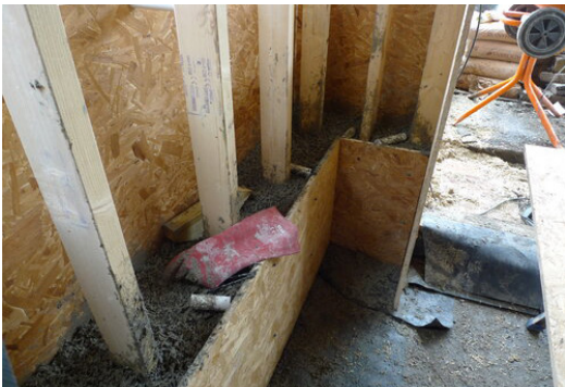
Image 14. Hand placing method
