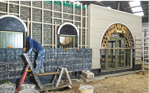
Image 30. Placing hempcrete on walls
