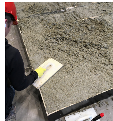
Spreading and tamping the mixture again, making it fit all around the frame.
