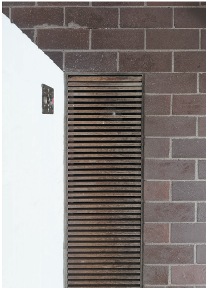
Wooden rods for heating shaft in the floor
