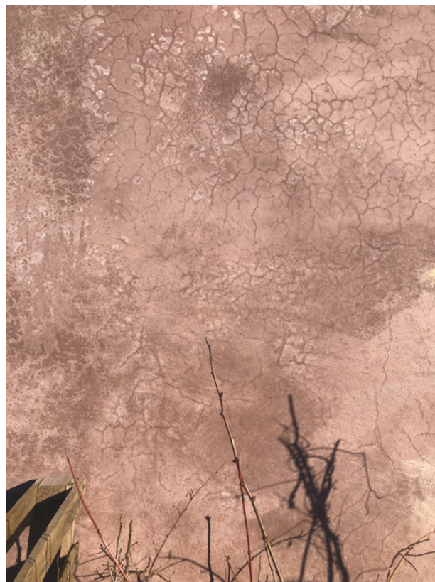
Illustration 6. Image showing cracks in clay plaster facade. Photo: Klara Moene-Omholt.
