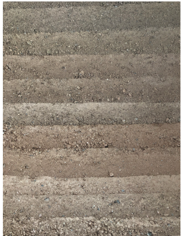
Illustration 28. Image rammed earth. Photo: Klara Moene-Omholt
