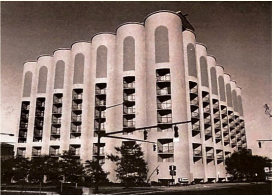
Example of adaptation from How Buildings Learn (1994). A former factory of the Quaker Oats Company was an appreciated landmark in the area. Because of its central location, the massive concrete structure was transformed into Quaker Hilton Hotel, allowed for the structure to be preserved yet economically viable. (Brand, 1994, p. 106) As Brand puts it: "ADAPTIVE USE opens minds to formerly unthinkable possibilities, such as converting concrete grain silos into a hotel" (Brand, 1994, p. 106)
