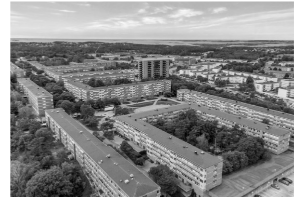
Figure 4.4: Open blocks, Västra Frölunda
