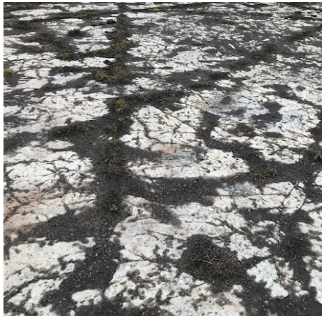
Fig 3.3 Visible limestone joints. (Own picture)
