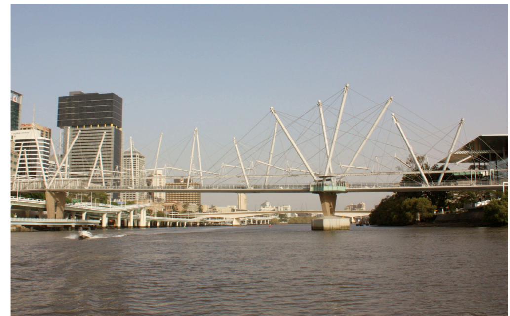
Figure 6: Kurilpa Bridge in Brisbane by Arup (2009).
