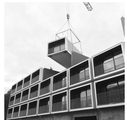
Fig 21. Snabba Hus pre-fabricated apartment
