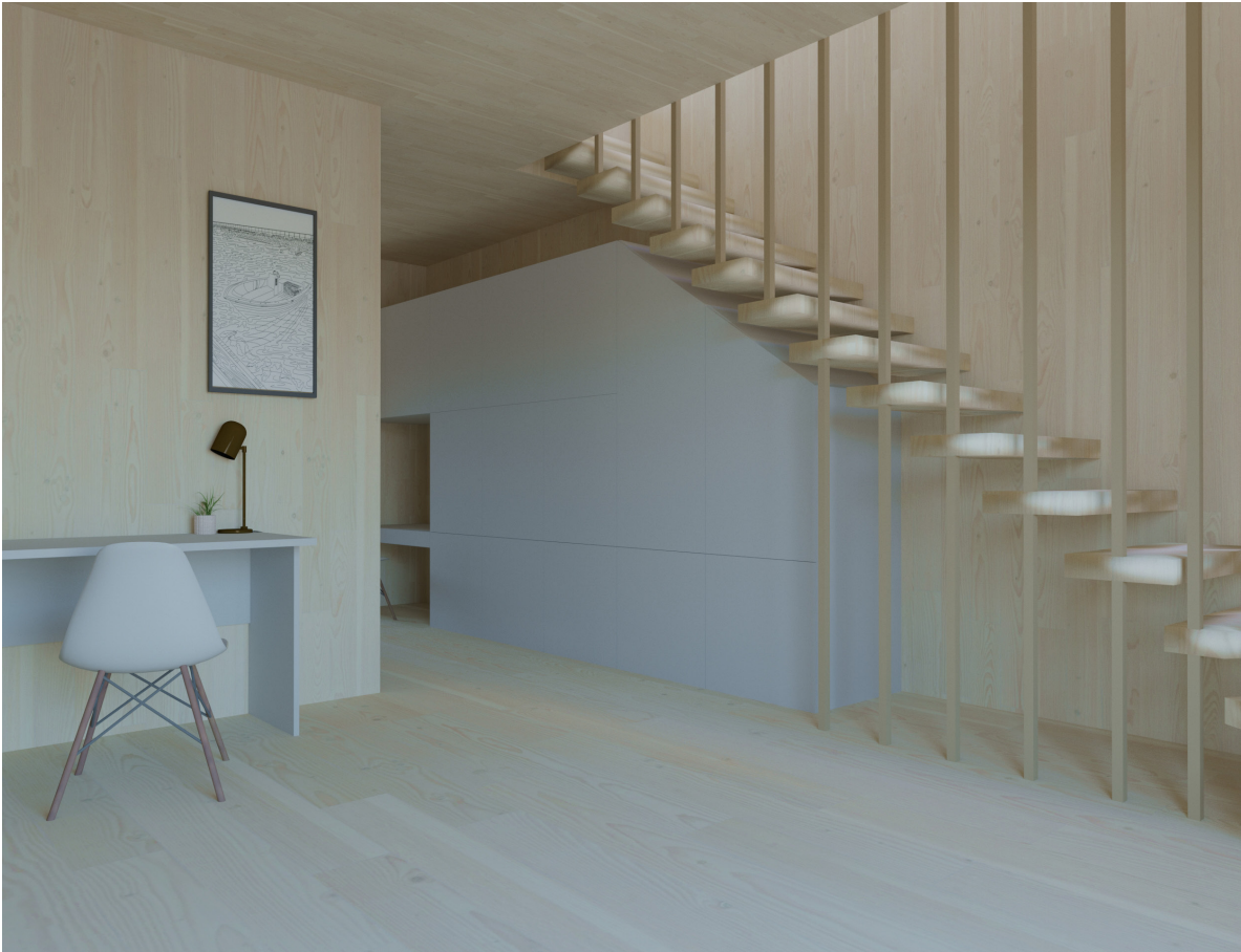
Interior of apartment CA CLT slabs are anchored into the wall to create the stair case
