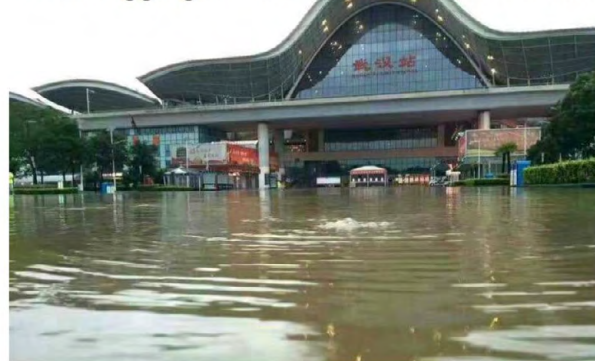
Waterlogging in 2016 : 28.37m (water level) & 229.1mm (in 14-hour)
