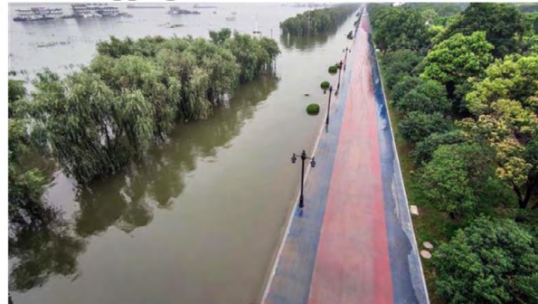
Waterlogging in 2020 : 28.77m (water level) & 165.9mm (in 24-hour)
