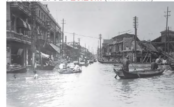
Flood in 1931 : 28.28m (water level)
