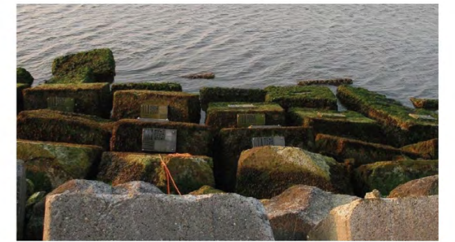
The seawall of Ellewoutsdijk (Netherlands)
