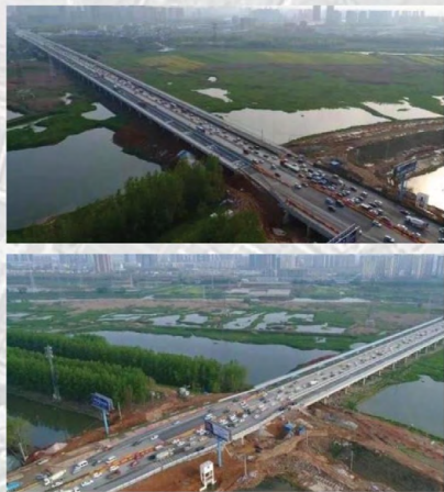
Daihuang Expressway Bridge of Fu River
