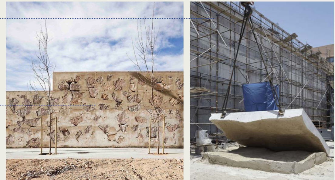
Fig 24 PARQUE VENECIA // HÉCTOR FERNÁNDEZ ELOR- ZA AND MANUEL FERNÁNDEZ RAMÍREZ Cyclopean wall/cyclopean con- crete, is a mix large stone blocks and concrete/cement. Traditionally "cyclopean refers to large blocks assembled with little or no mortar.
