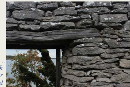
Stone structure in change. Masonry limestone structure where previous opening is filled with drystoned limsetones, Gotland
