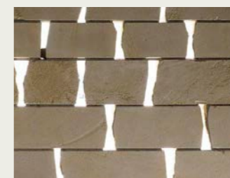
II: Guest houses: The stone as craft. Stereotomy and transparency. Stonemasonry techniques as detail.
