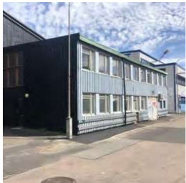
The small office building
