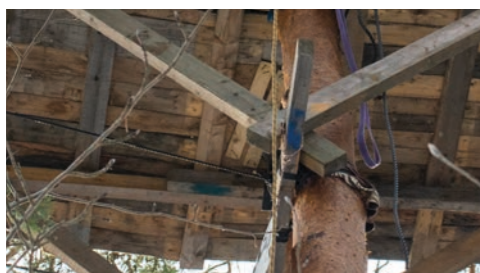
Photograph: Construction detail treehouse Blodstenskogen
