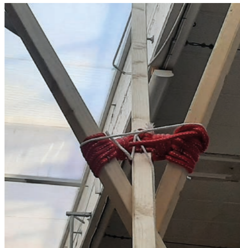
Photograph: How a tripod is tied
