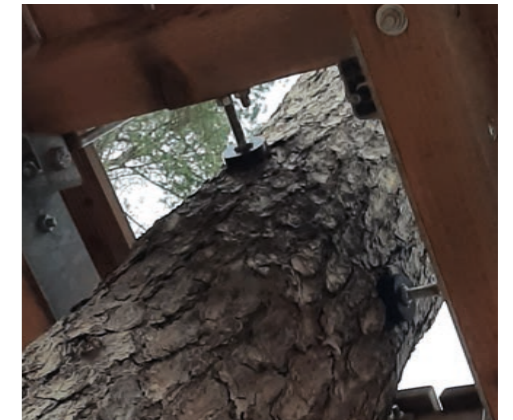
Photograph: Small platform support around stem
