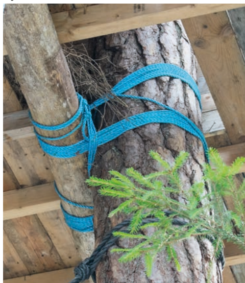
Photograph: Construction detail treehouse Blodstenskogen
