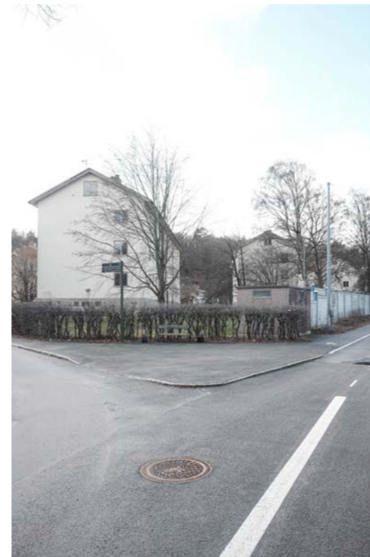
The opening in the sound barrier is right at the beginning of Kv Törnrosen. Here you meet the short sides of the slats, which are separated by a
