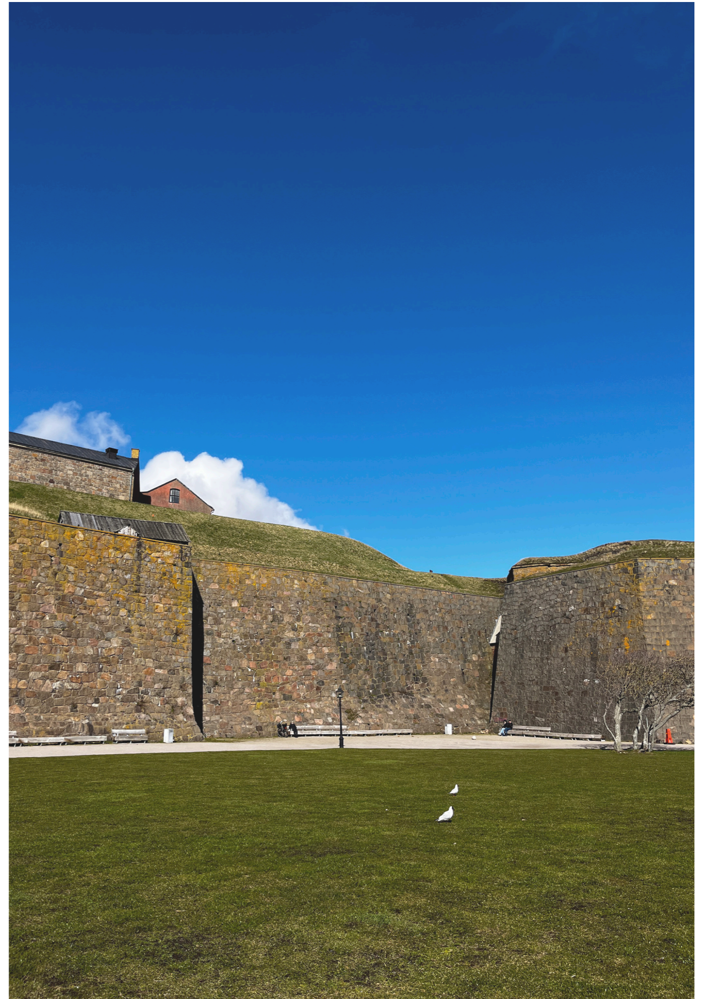
Photograph of the south side of the fortress on March 27, 2023.
