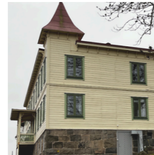
Wood facade & stone base
