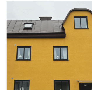
Render & metal sheet roof
