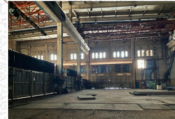
image 26-36. on-site pictures. Photos: Y. Chen
