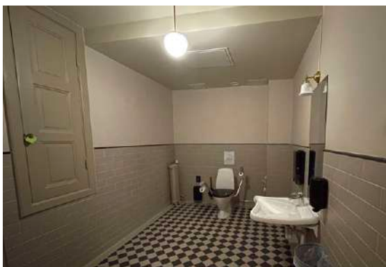
Image 34. The addition of an RWC after the renovation in 2015.
