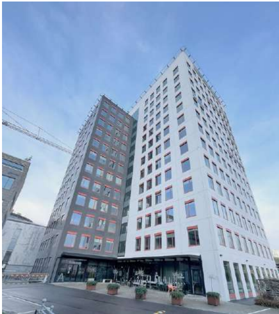
Image 11. (a) Office building, where PEAB's office is located.
