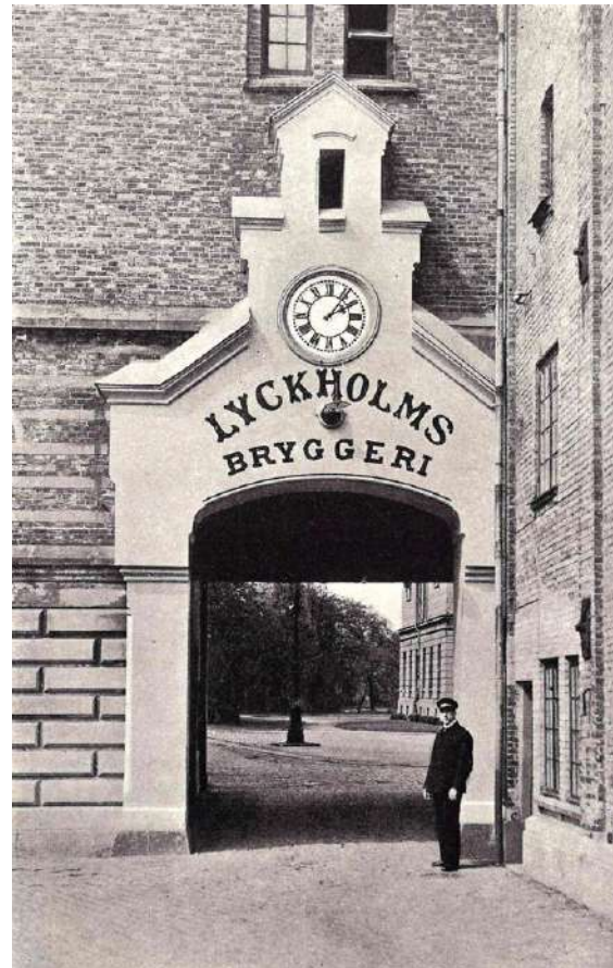
Image 1. The main entrance where leads to the manager's house.
