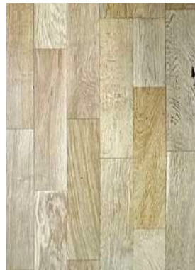
Image 36. The repaired wooden floor.
