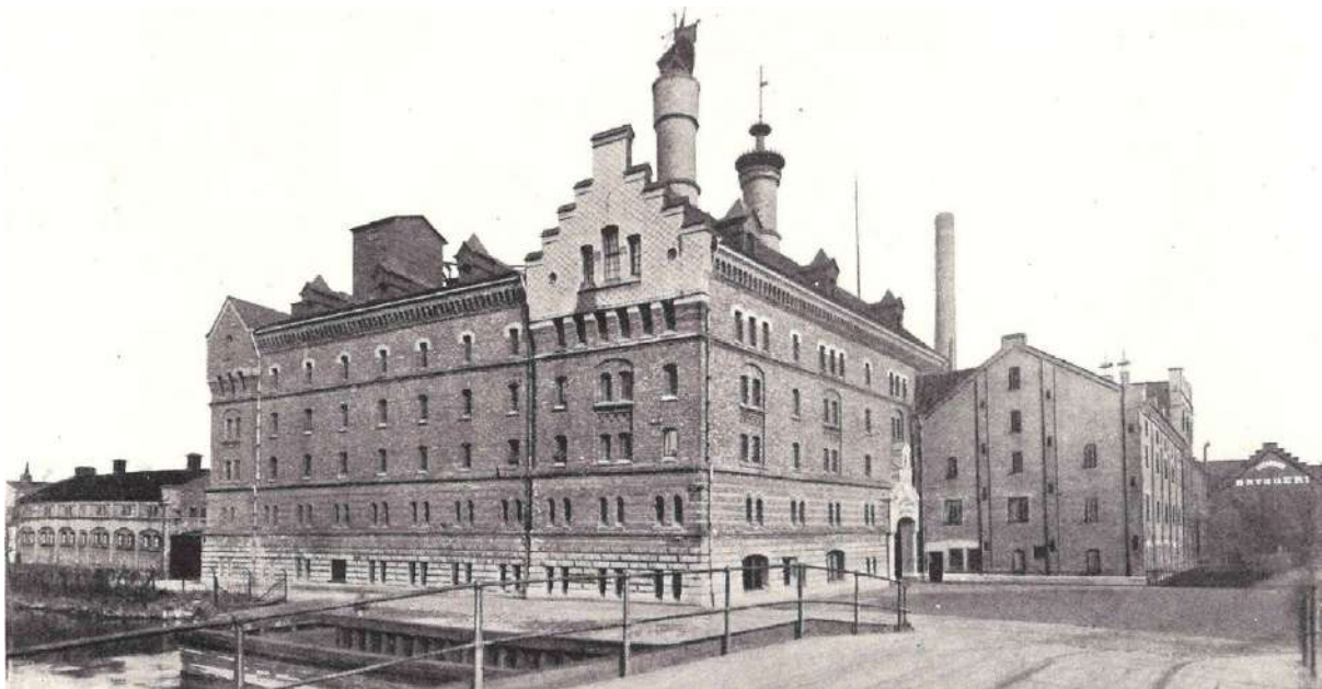
Image 3. Scene from the bridge on Möndalsån.
