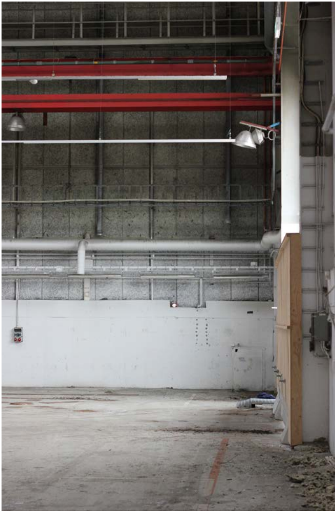
Poetic, northern light entering in a corner of the building.
