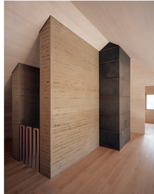
Figure 13: House K's interior showing the chimney of rammed earth (Arch daily, 2023).
