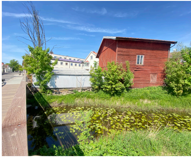
Figure 35: View from the east towards the tannery with Söderån in front.
