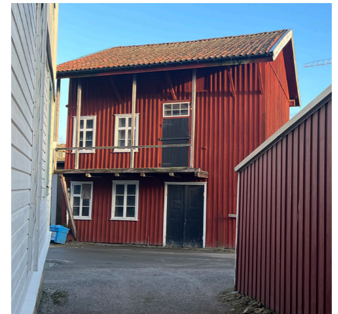
Figure 43: The tannery building that is left today.
